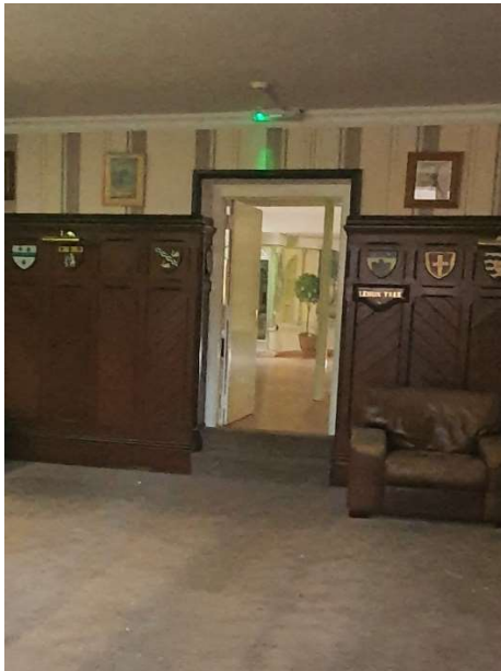
Existing Opening in the Bar Area
