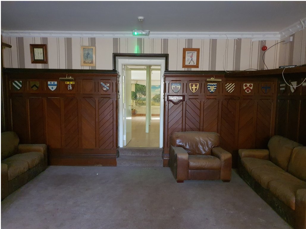
View of the Existing Opening with Timber Panelling
