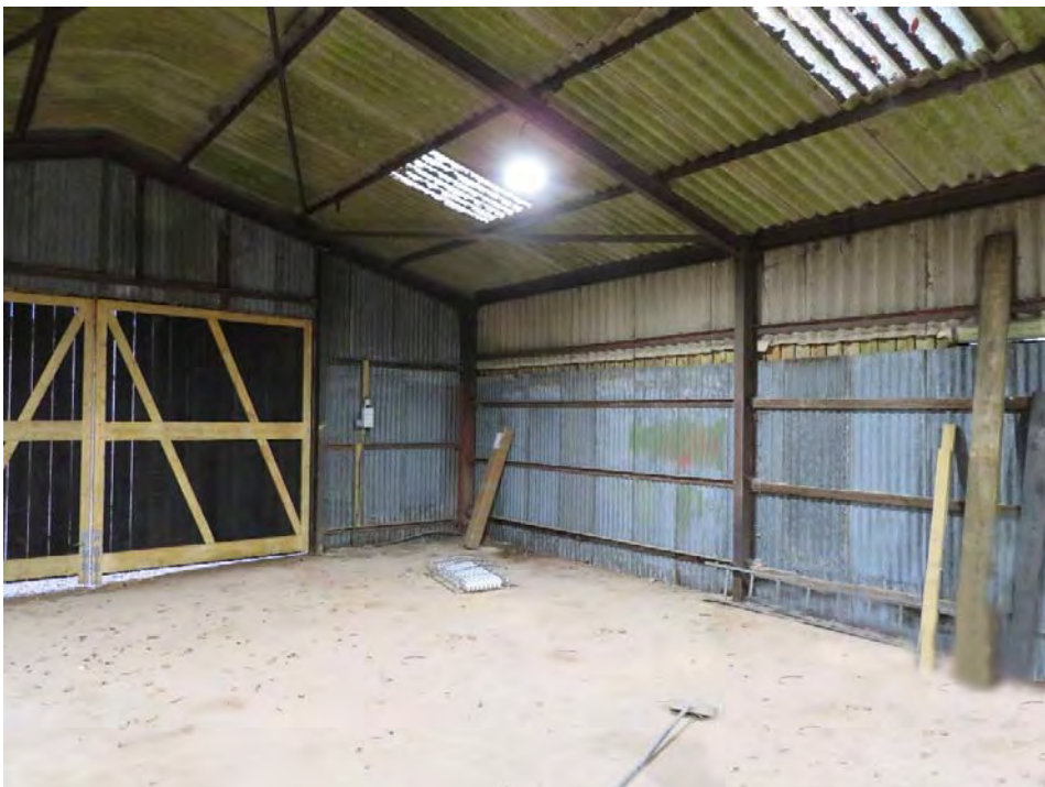
Photograph 8: Partial internal view of barn - nearest road.
