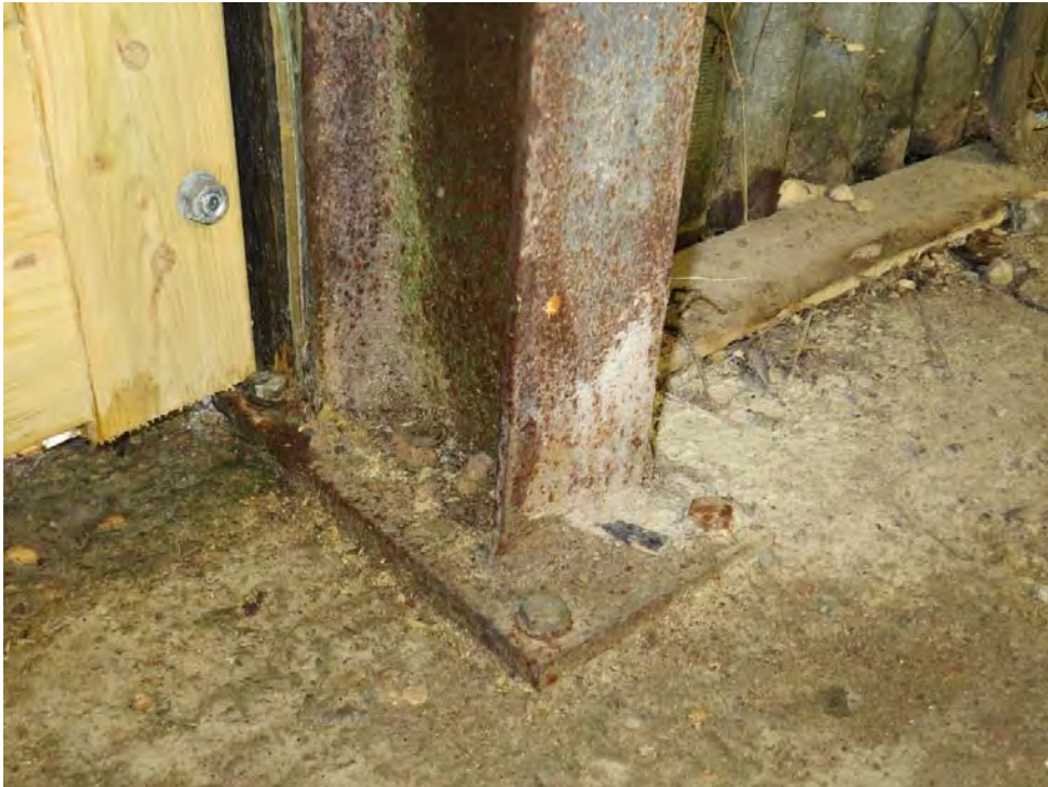
Photograph 5: Columns adjacent door built directly off slab.
