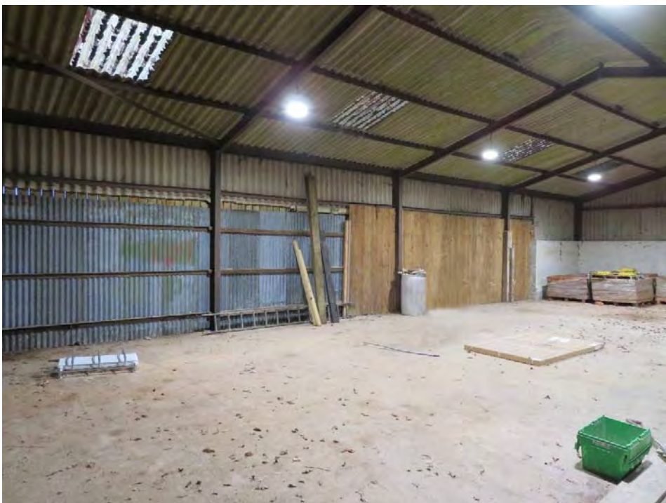
Photograph 10: Partial internal view of barn - nearest road.
