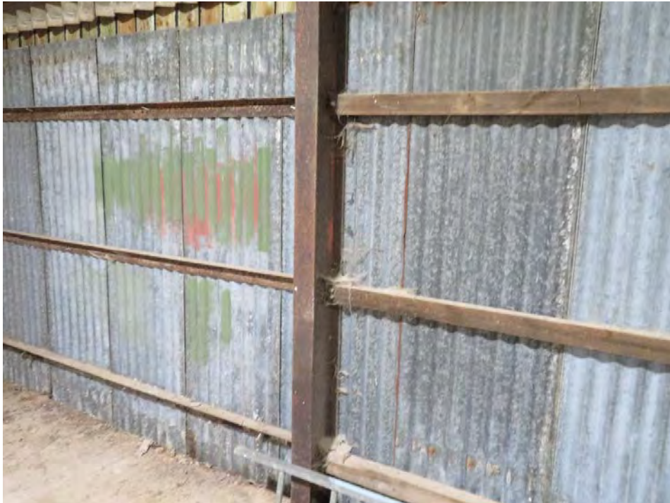
Photograph 11: Steel rail replaced with timber sections.
