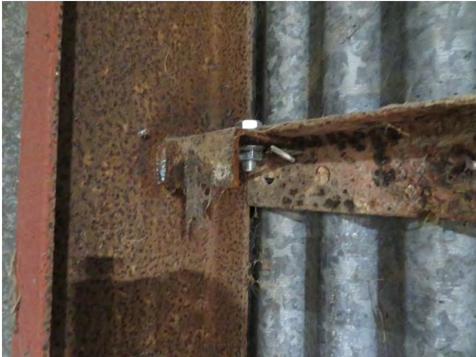
Photograph 13: New bolts at rail/column connection.
