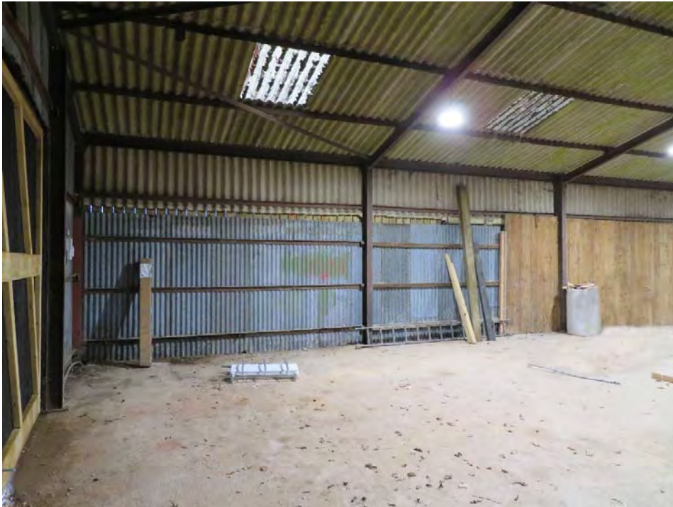
Photograph 9: Partial internal view of barn - nearest road.
