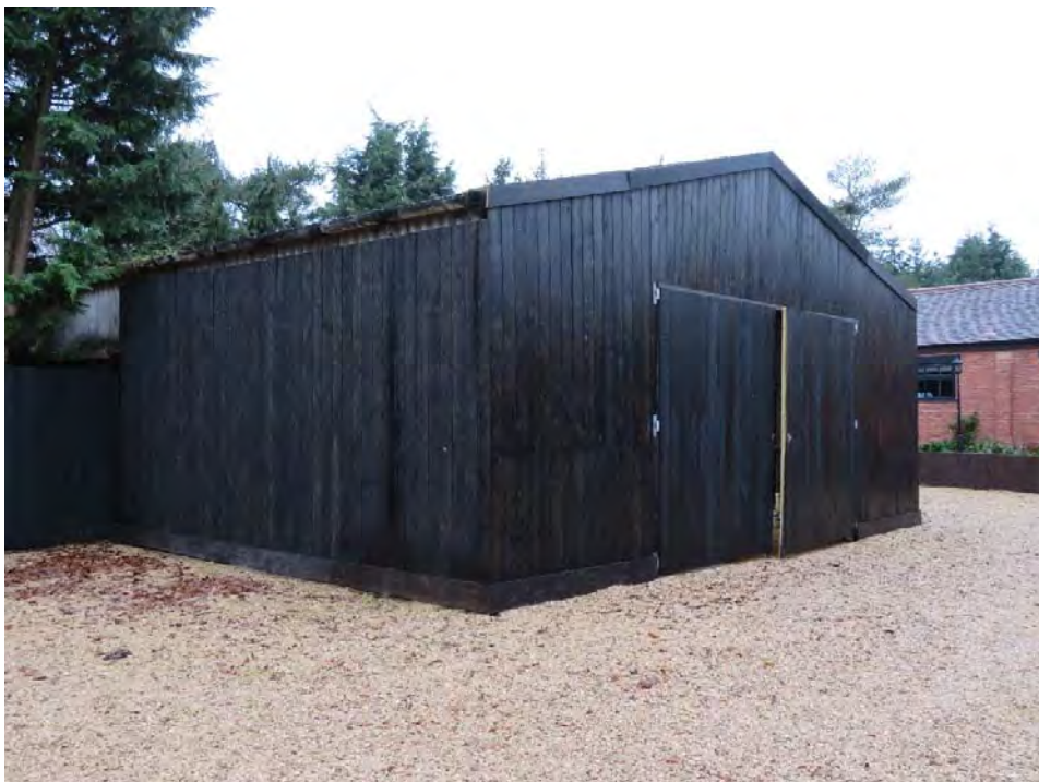
Photograph 2: Front/Side elevation (nearest road).
