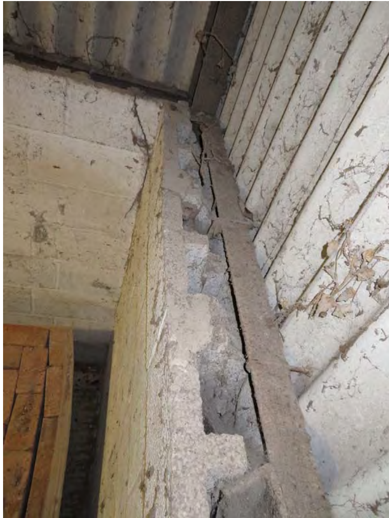
Photograph 16: 215mm thick Hollow blockwork wall to rear and side of barn.
