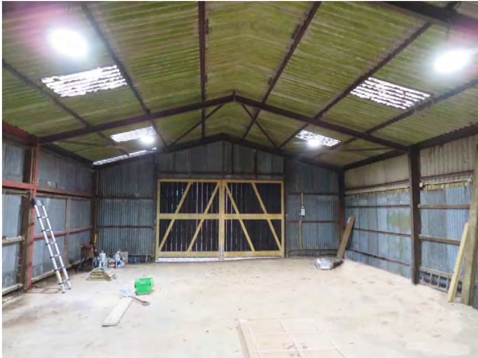
Photograph 3: Wind girder present in first bay.
