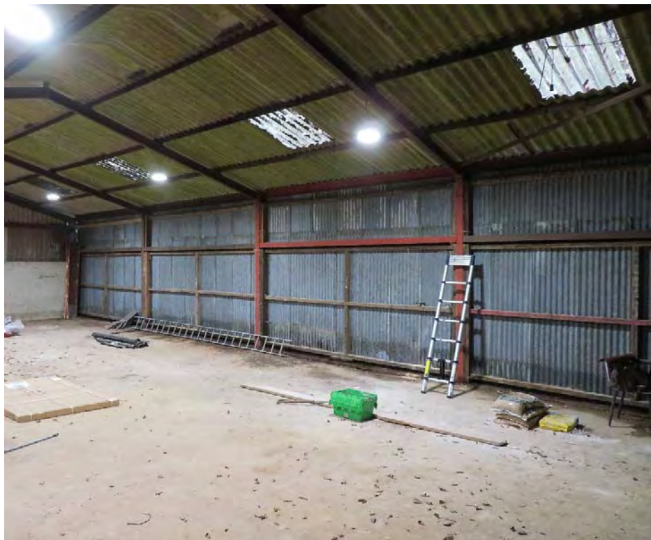
Photograph 14: Partial internal view of barn – nearest dwelling.
