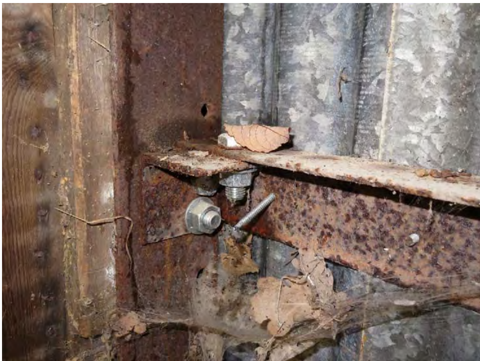
Photograph 12: New bolts at rail/column connection.
