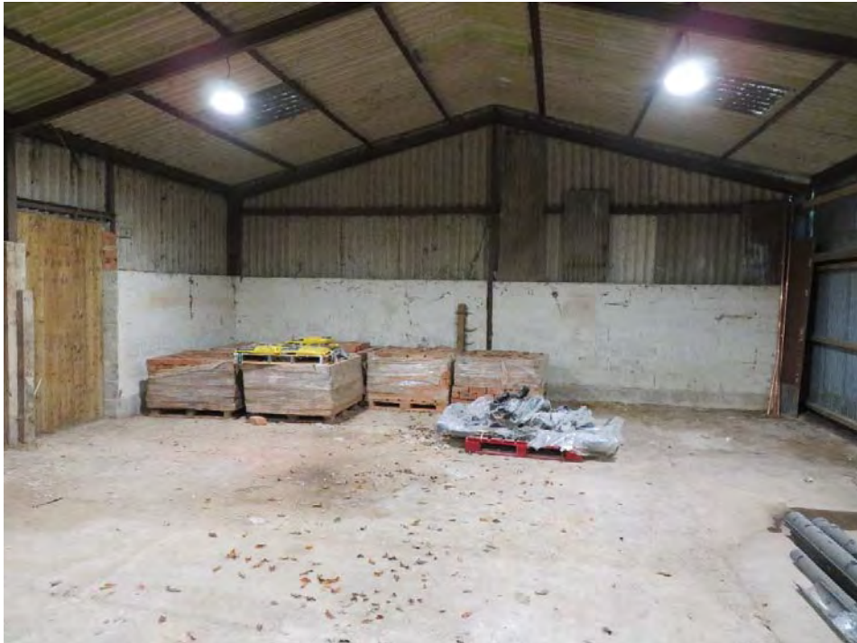
Photograph 15: 215mm thick Hollow blockwork wall to rear and side of barn.
