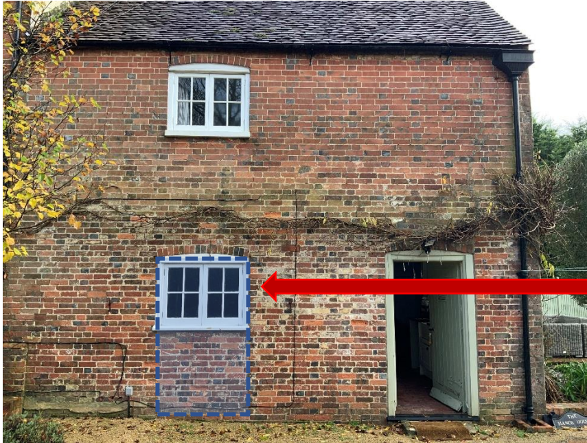
External view of existing annex living room window – to be replaced with full length timber frame double doors, the width of the structural opening is to remain the same.
