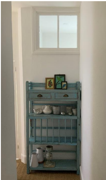
View of existing internal bathroom window from the landing – to be blocked up
