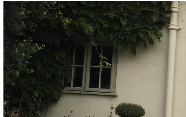
External view of existing annex kitchen window - to be widened
