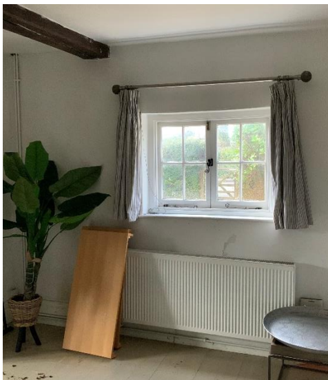
Internal view of existing annex living room window.
