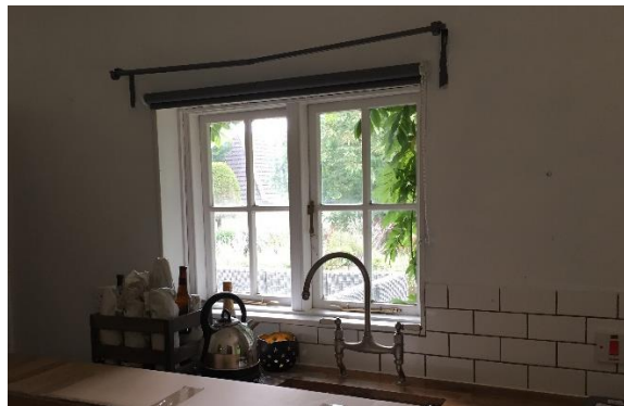
Interior view of existing annex kitchen window - to be widened
