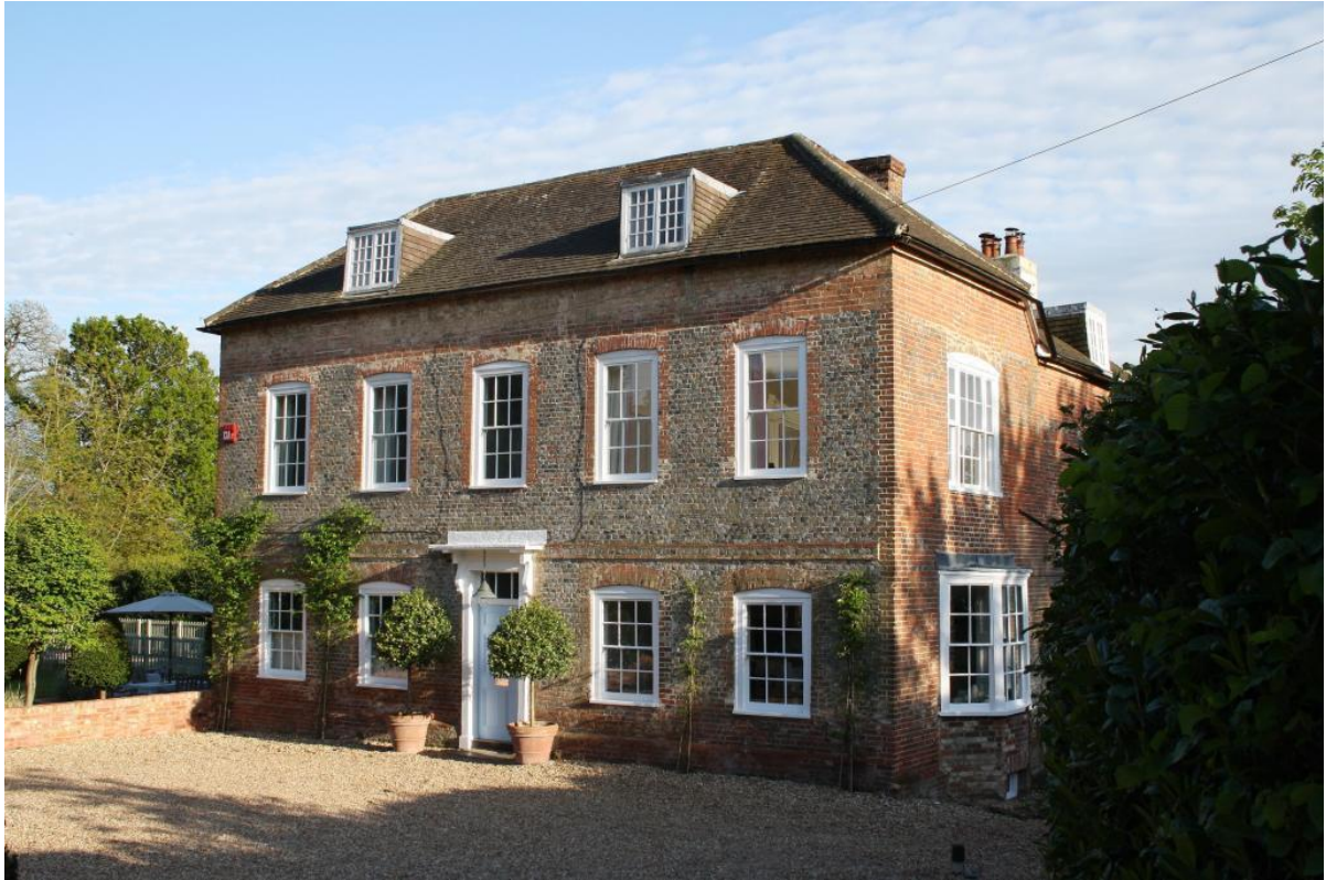
Front of dwelling – North Elevation
