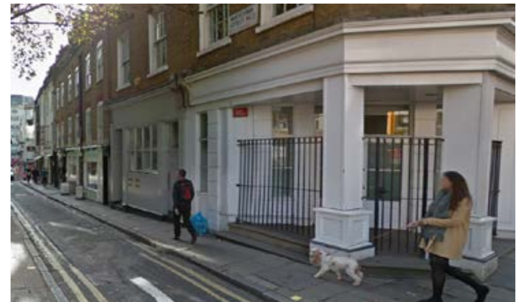
View of facade along Whitcomb Street
