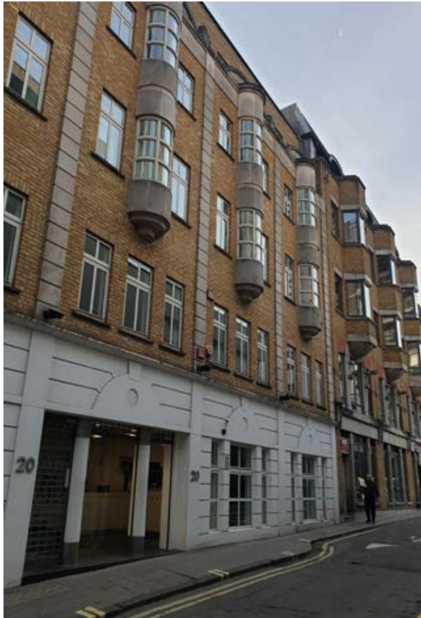
View of front facade
