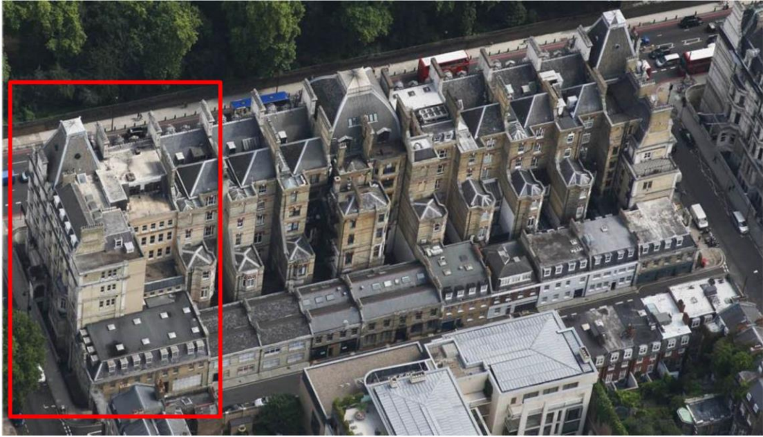
Figure 3.1 Aerial View showing rear of terrace to Headfort Place.
