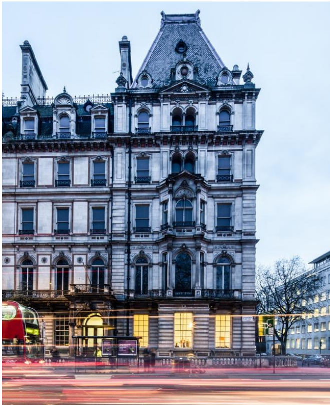
Figure 1.1 – View of façade from Grosvenor Place
