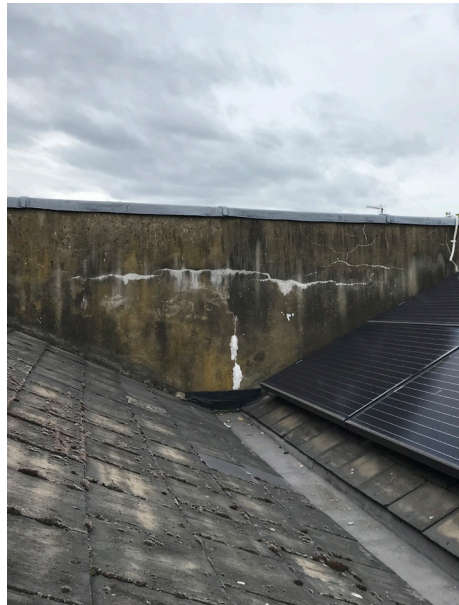
Existing slate butterfly roof set behind parapet
