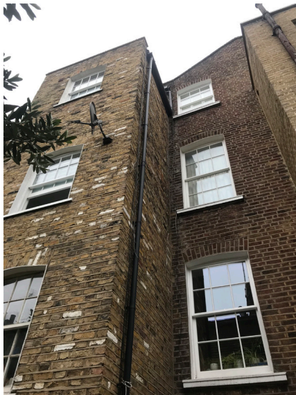
Existing rear elevation above lower ground floor level
