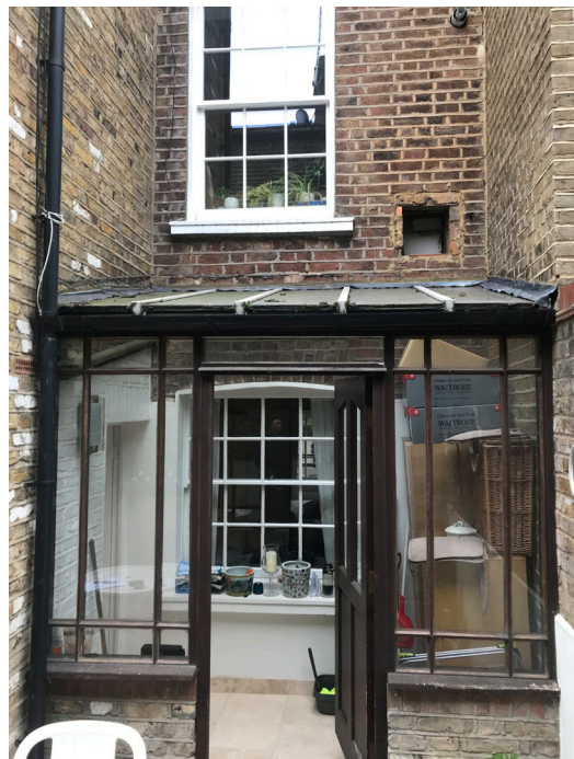
Existing rear infill extension
