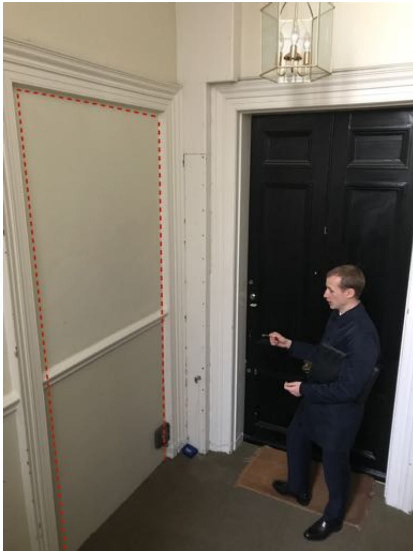
IMAGE 01 - BUILDING N.42 RED DOTTED LINE ON PICTURE INDICATING NEW ENTRANCE DOOR TO FLAT 1 EXISTING ENTRANCE DOOR (BLACK PAINTED) TO BE KEPT IN SITU
