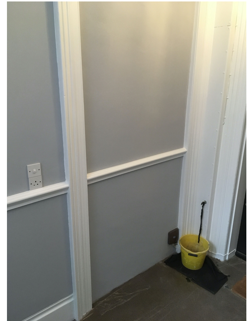
IMAGE 03 - BUILDING N.42 EXISTING ARCHITRAVE TO BE KEPT IN SITU.
