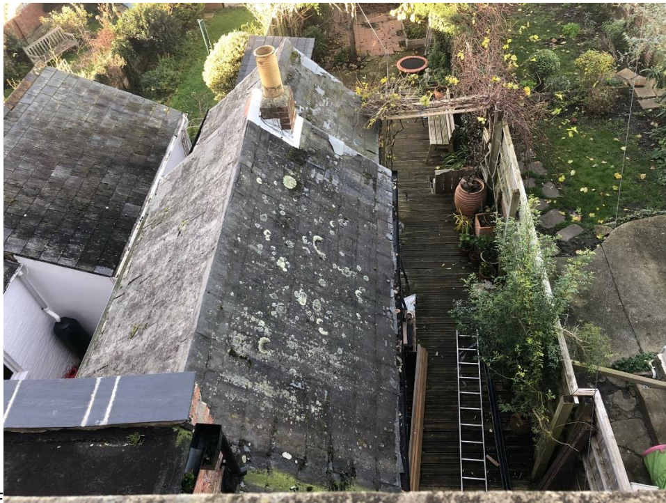
Existing side return roof.
