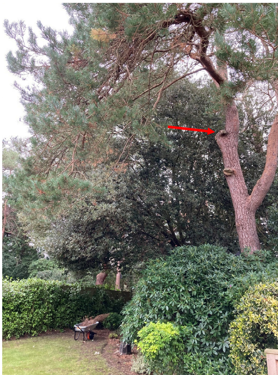
Pic.4 – Form of T3 Decayed pruning wound indicated with arrow
