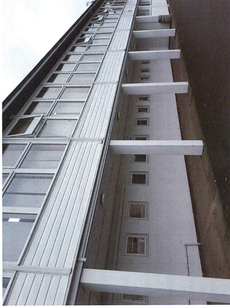
Rear of the Derry House Building
