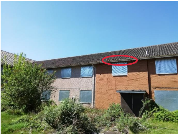
Figure 6 – South-eastern aspect of two-storey section and known emergence point (x1)
