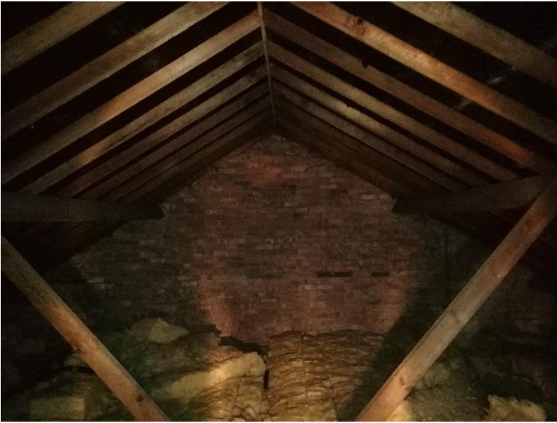
Figure 3 – Interior of roof void
