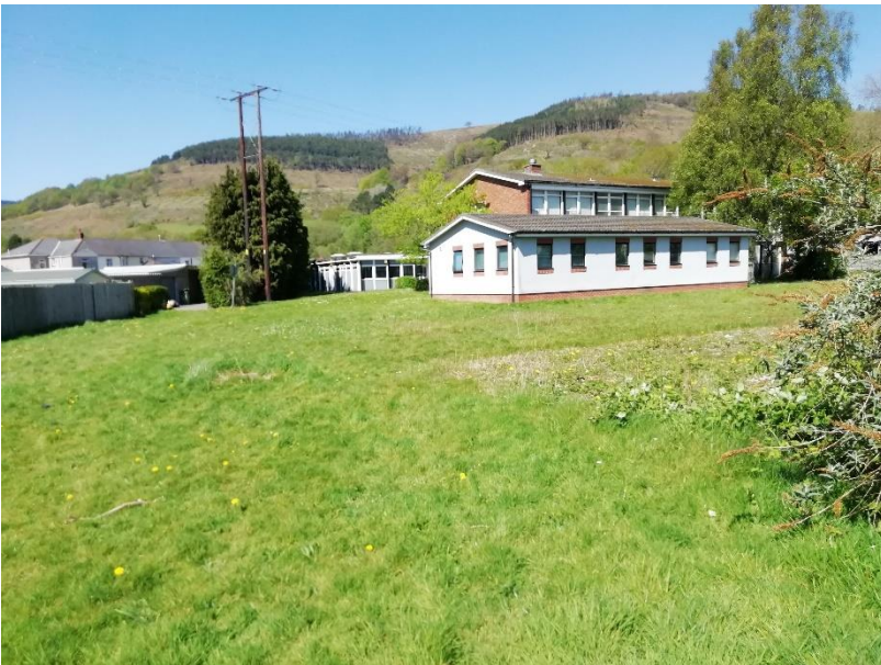
Figure 8 – View to north (offsite)
