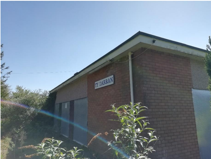
Figure 11 – Eastern aspect of flat-roofed section
