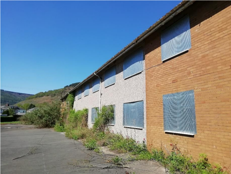
Figure 7 – Western aspect of building
