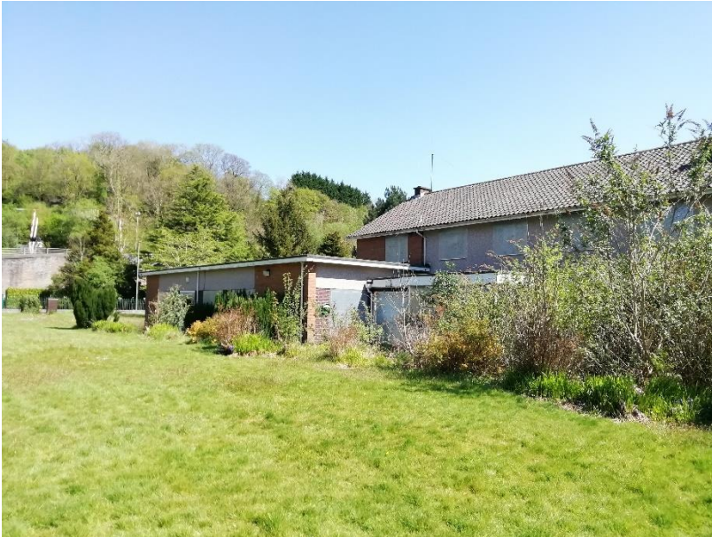
Figure 9 – View towards eastern end of northern elevation
