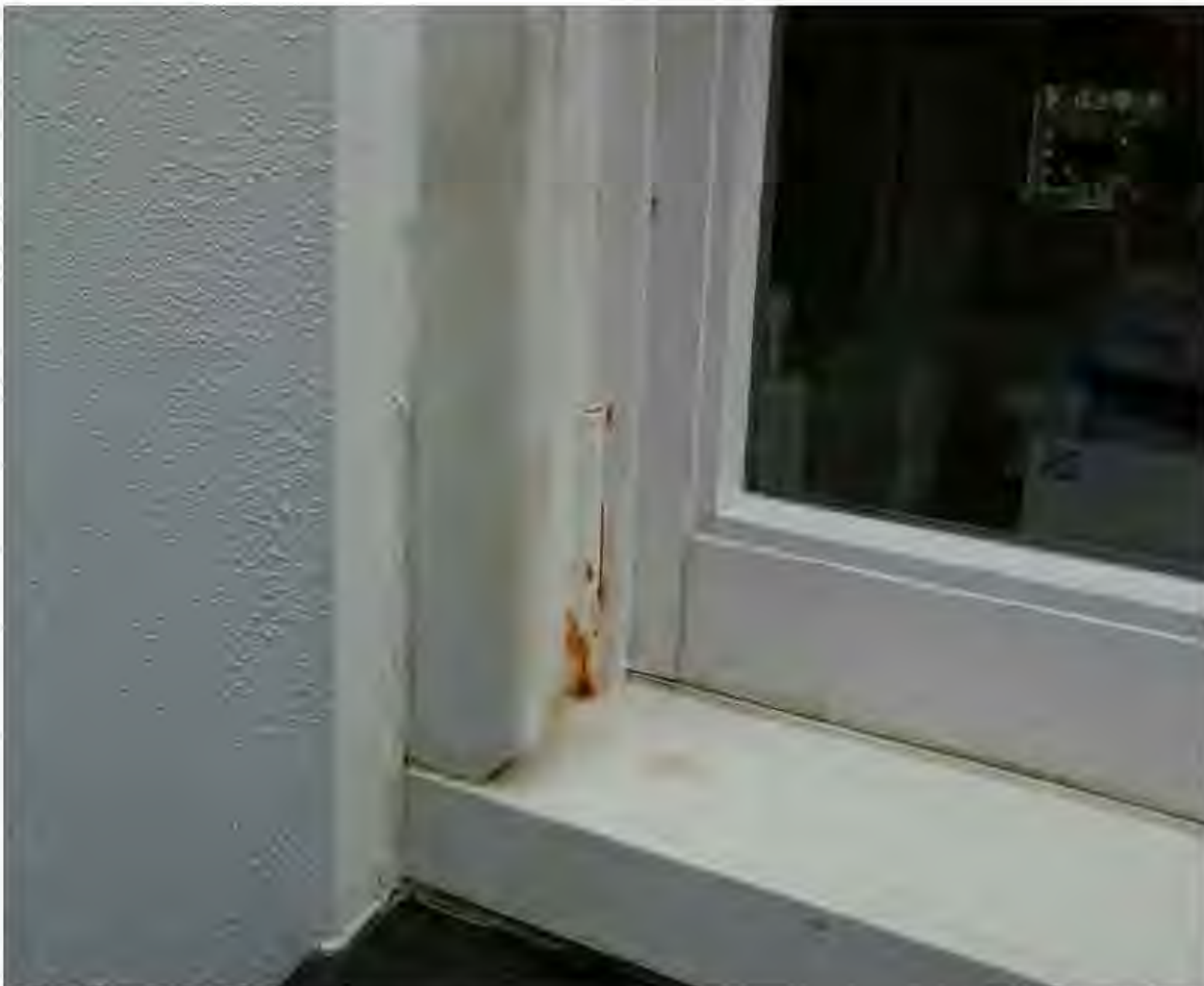
Example of Previous Window Repair
