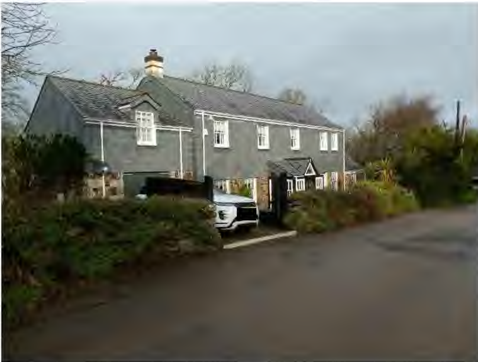
Existing Front Elevation to Highway (Looking North)
