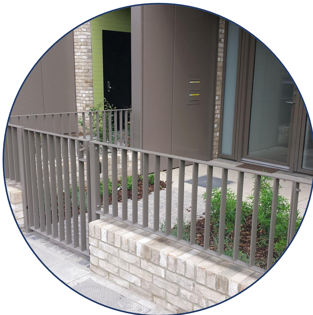
Front garden & Entrance Railings Aluminium flat bar to top of railings with flat bar vertical rails at 75mm centres below. Colour RAL 7034 - Yellow Grey
