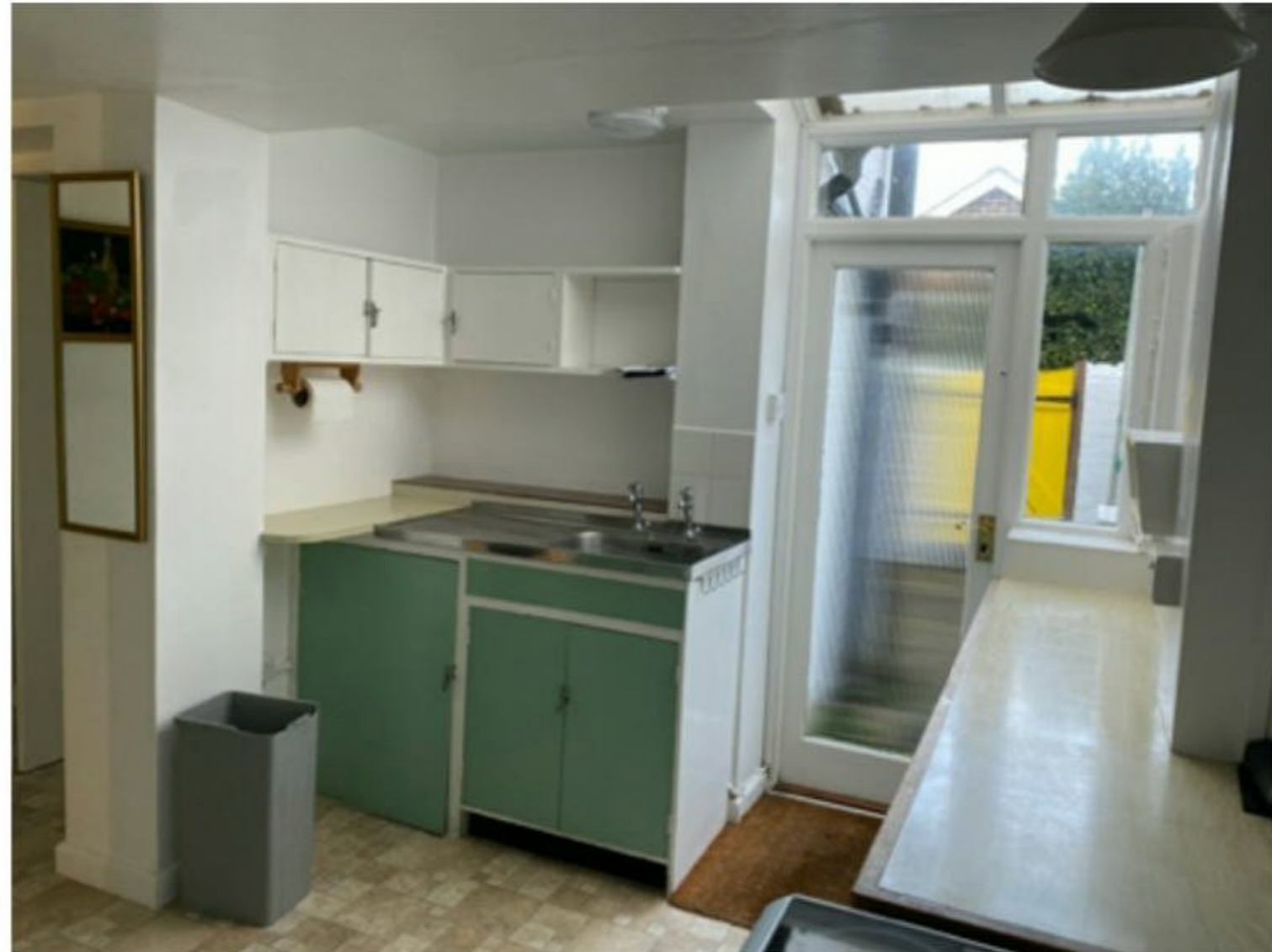
Above: View of the current kitchen layout within the 20 th Century rear extension
