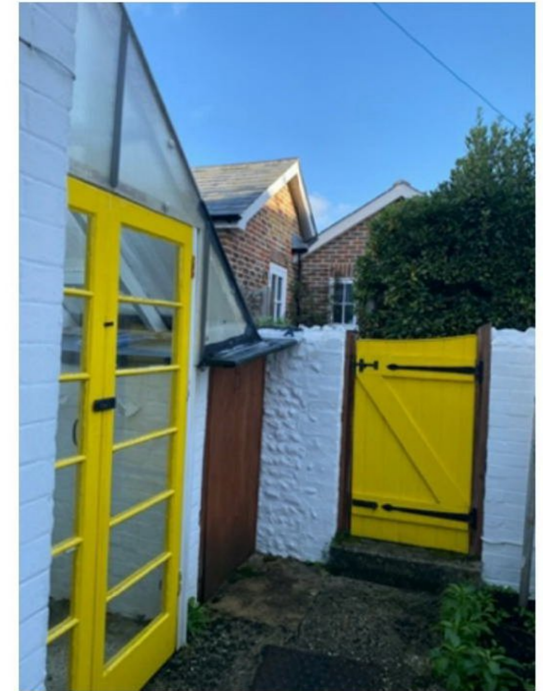
Above: Side-view of the rear elevation lean-to and rear wall.
