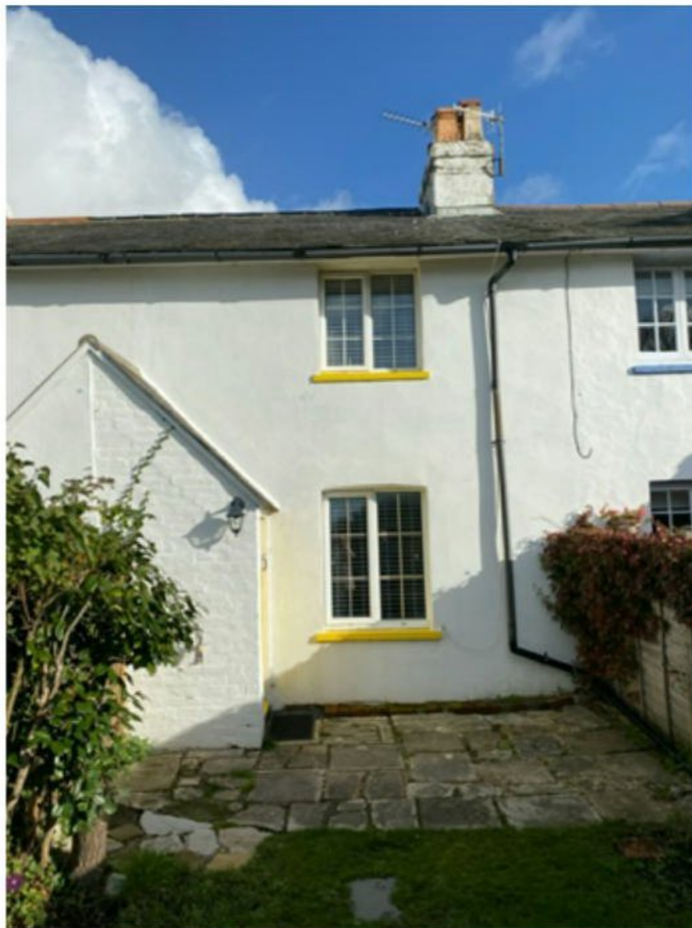
Above: Front elevation of the Cottage overlooking the harbour
