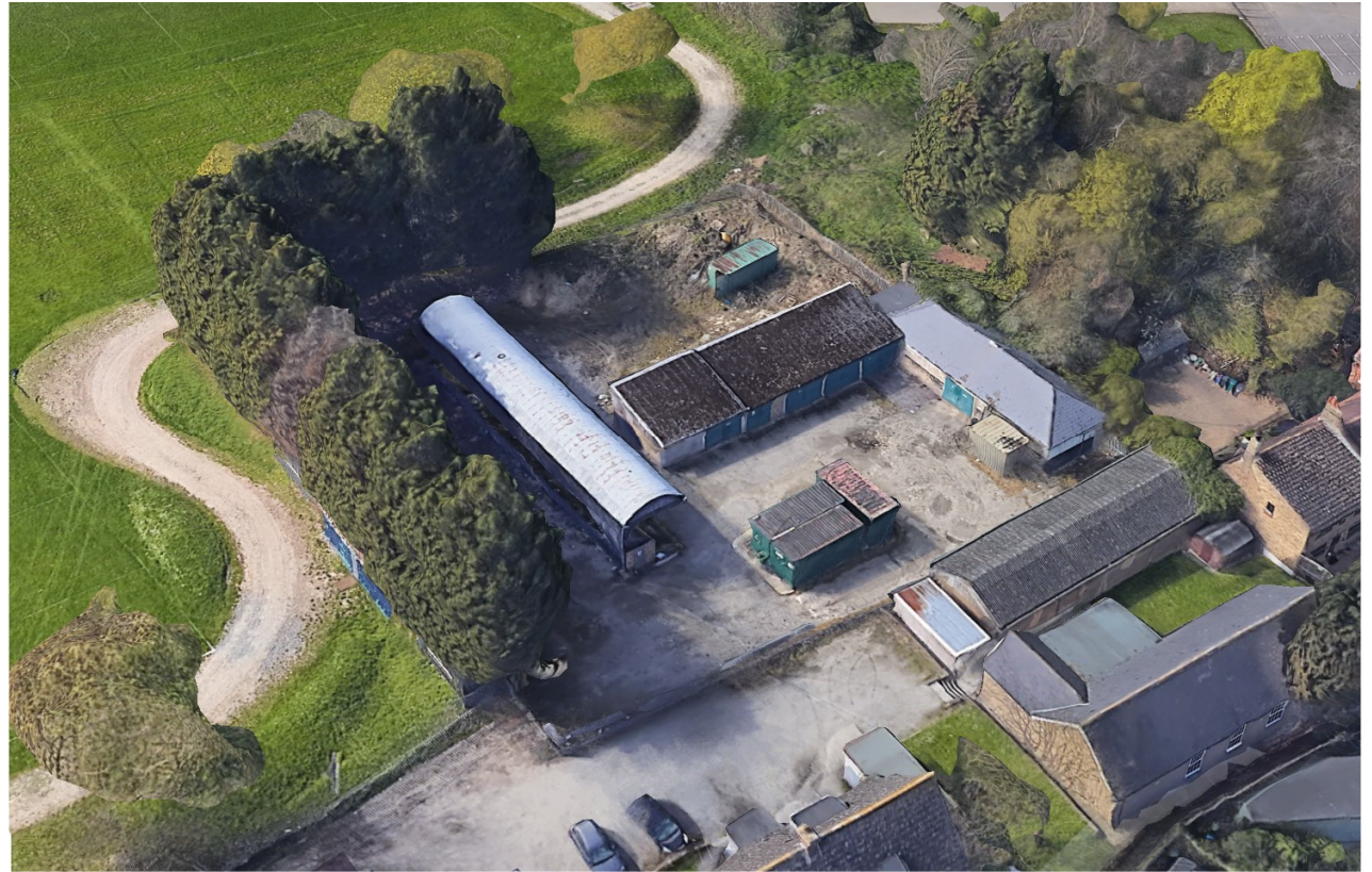
Site Aerial View
