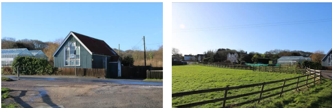
Buildings to the west separated by the public highway
