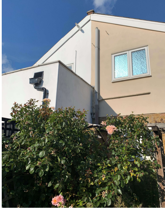
Photo 03: Rear view on the existing extension at Park road number 39.
