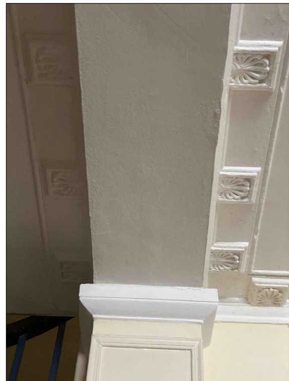
Existing GF cornice to match (extend in Lobby G-02 and install in Seating room G-03)
