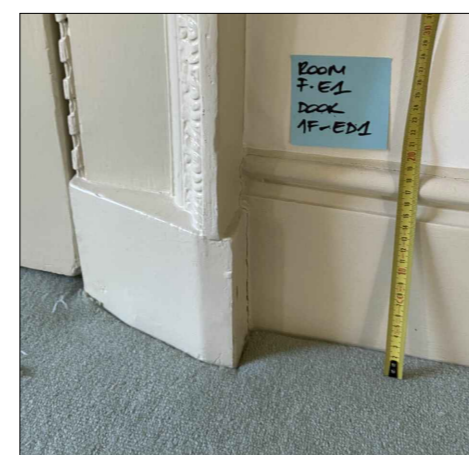
Existing 1F Skirting (Living room F-01) to be fully refurbished
