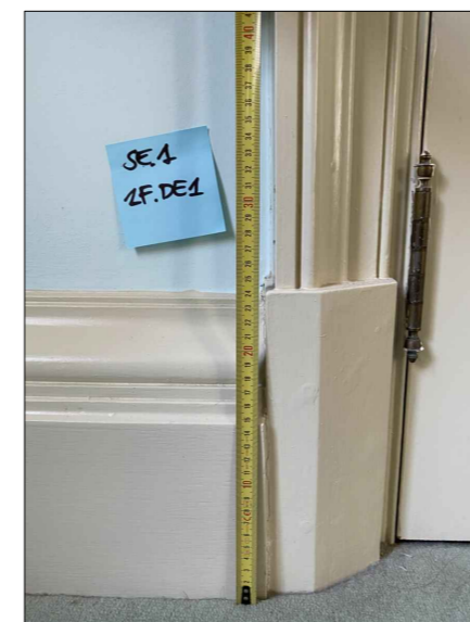
Existing 2F skirting (Master Bedroom SE1) to be fully refurbished
