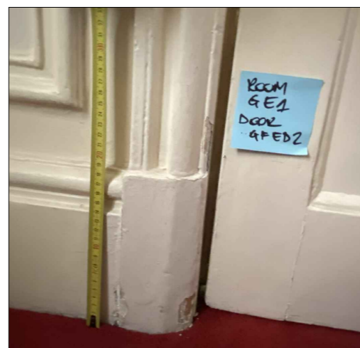
Existing GF skirting (Dining room G01) to be fully refurbished
