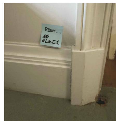
Existing LGF skirting (Bedroom 1 LG.E1) to match
