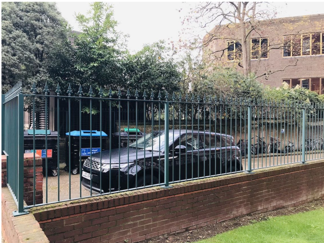
View of site from Finchley Place, plant to be concealed behind site boundary fencing, perimeter trees and landscaping
