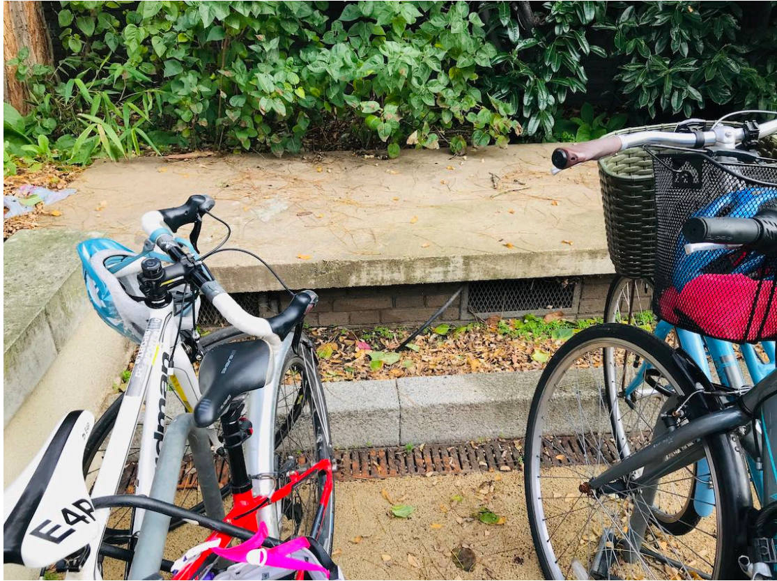
Detail of existing upstand vent, with wall and rc concrete slab
