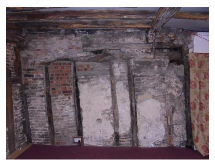
The above photograph shows the existing wall with apertures that are to be repaired with tile insert utilising lime mortar to bond the tiles together. See drawing 20/103/6
