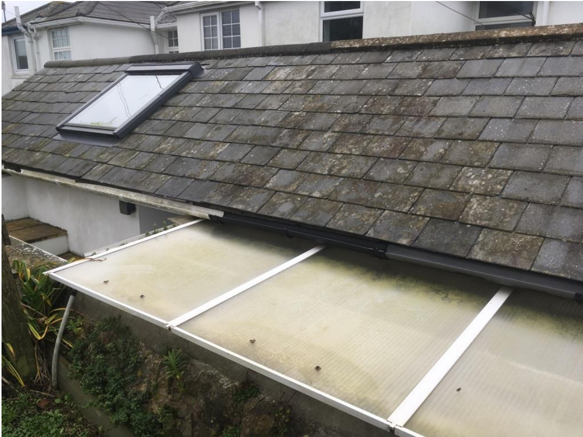
Boot room roof and roof to adjoining property.
