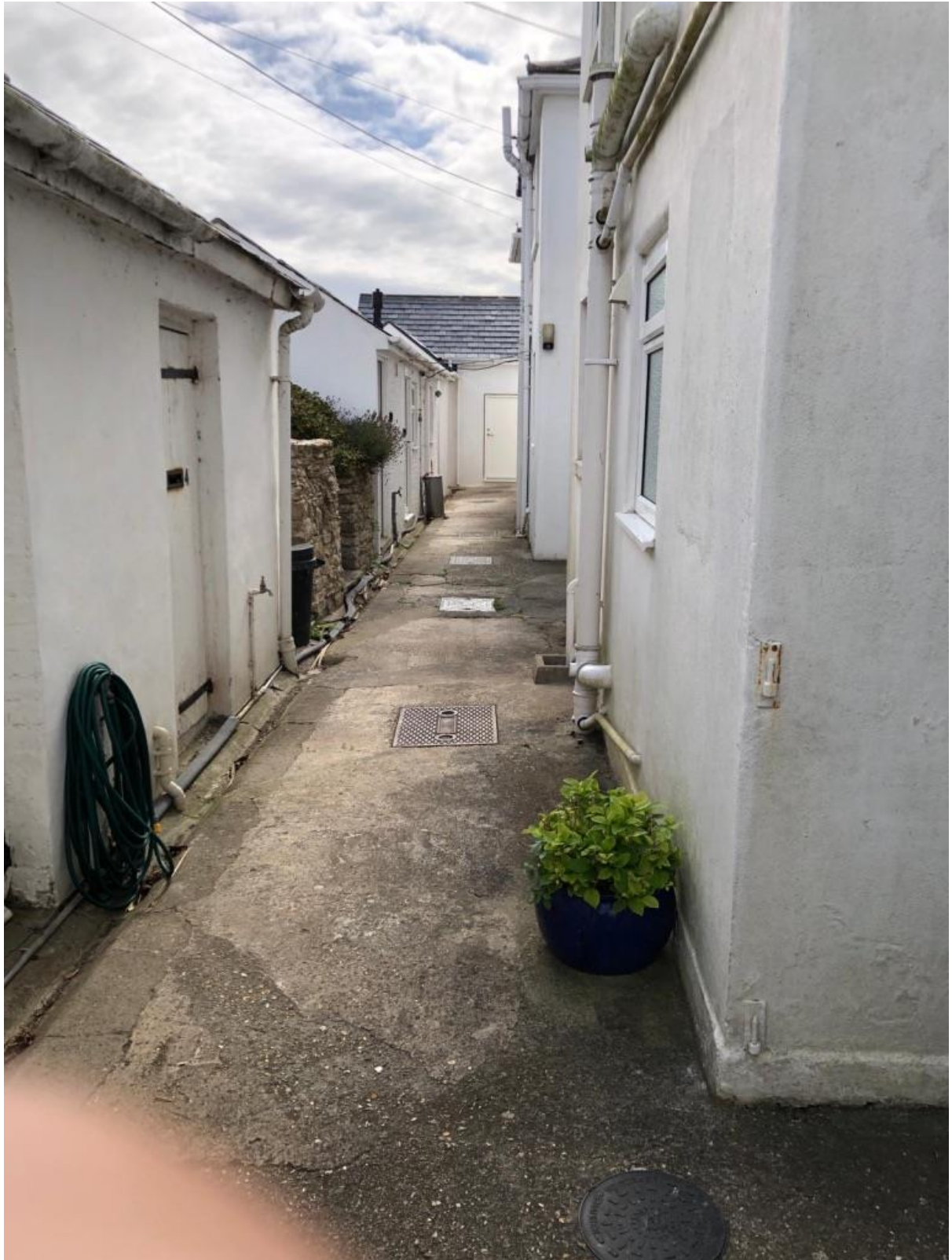
Communal path to the north side of Coastguard Cottages looking east from 6 Coastguard Cottages
