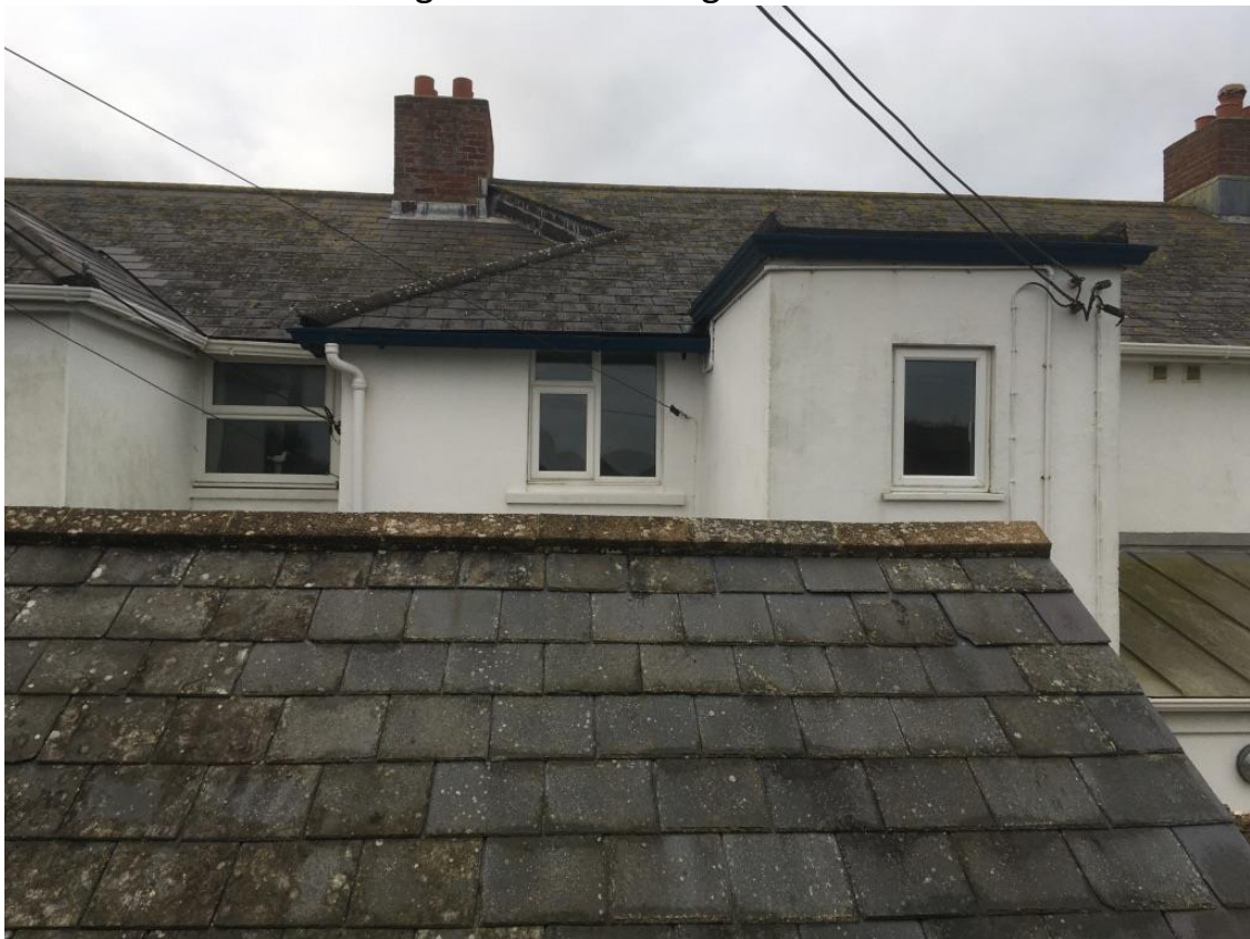
North facing roofs 6 Coastguards Cottage.
