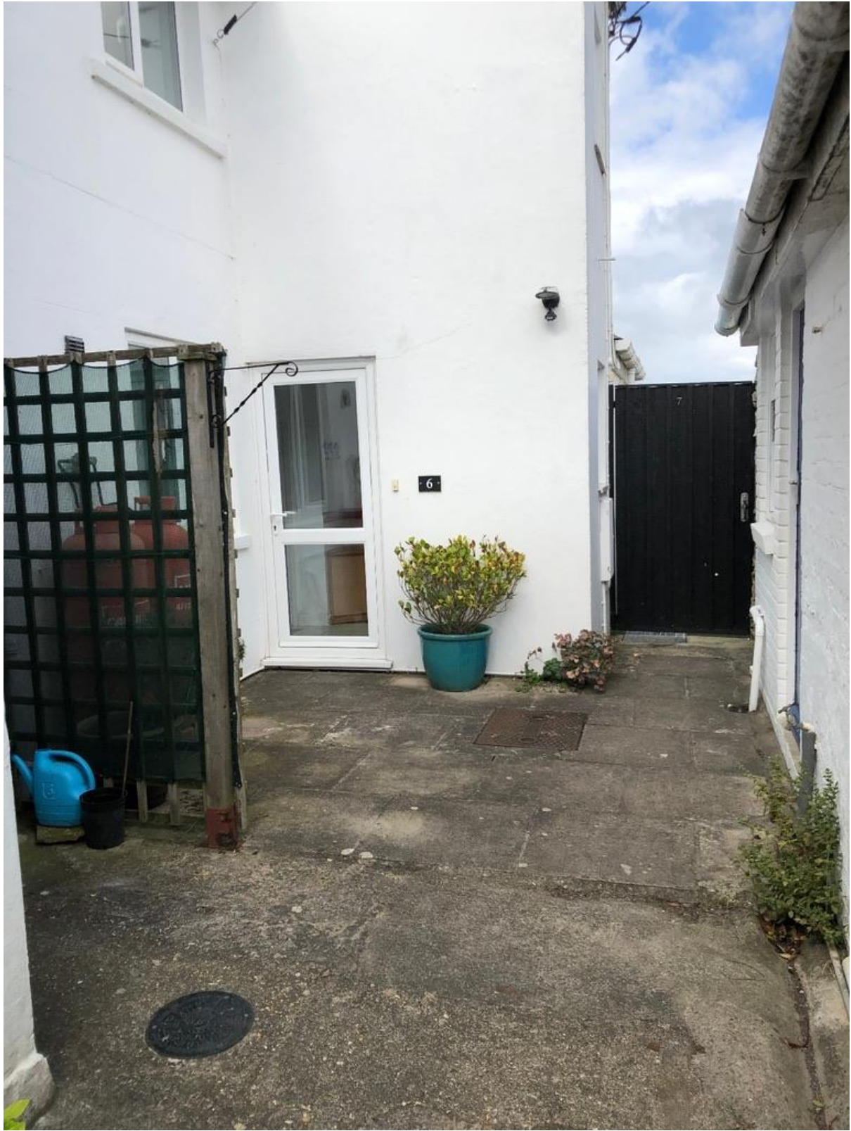
Looking west towards 6 Coastguard Cottage, with house on the left and boot room on the right and gate to 7 Coastguard Cottage.
