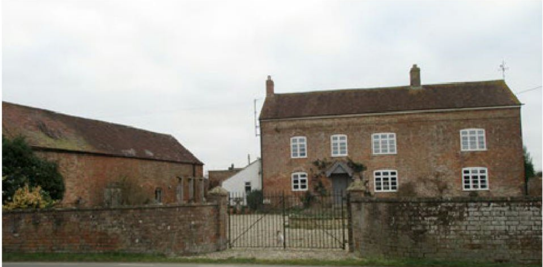
West elevation of Saul Farm House (20)
