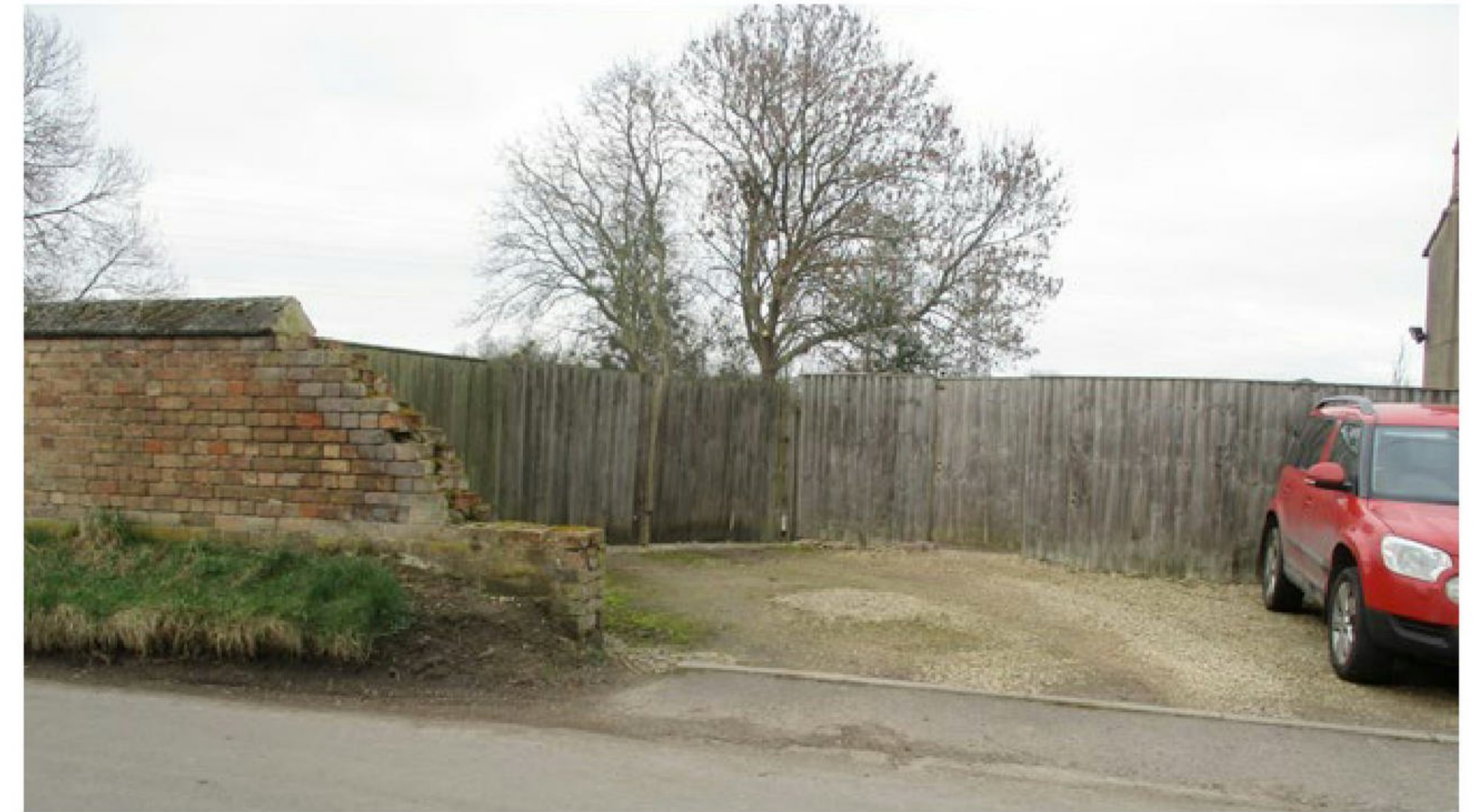
Existing vehicular parking for Lion House and access to proposal site. (08)
