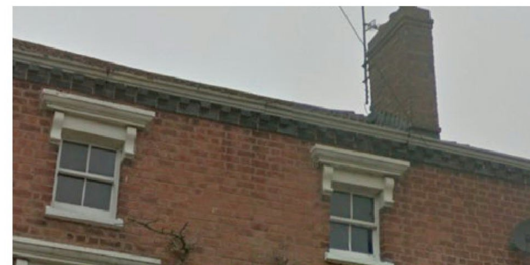
Window head detail, red brick chimney and brick coursing detail on neighbour (46)
