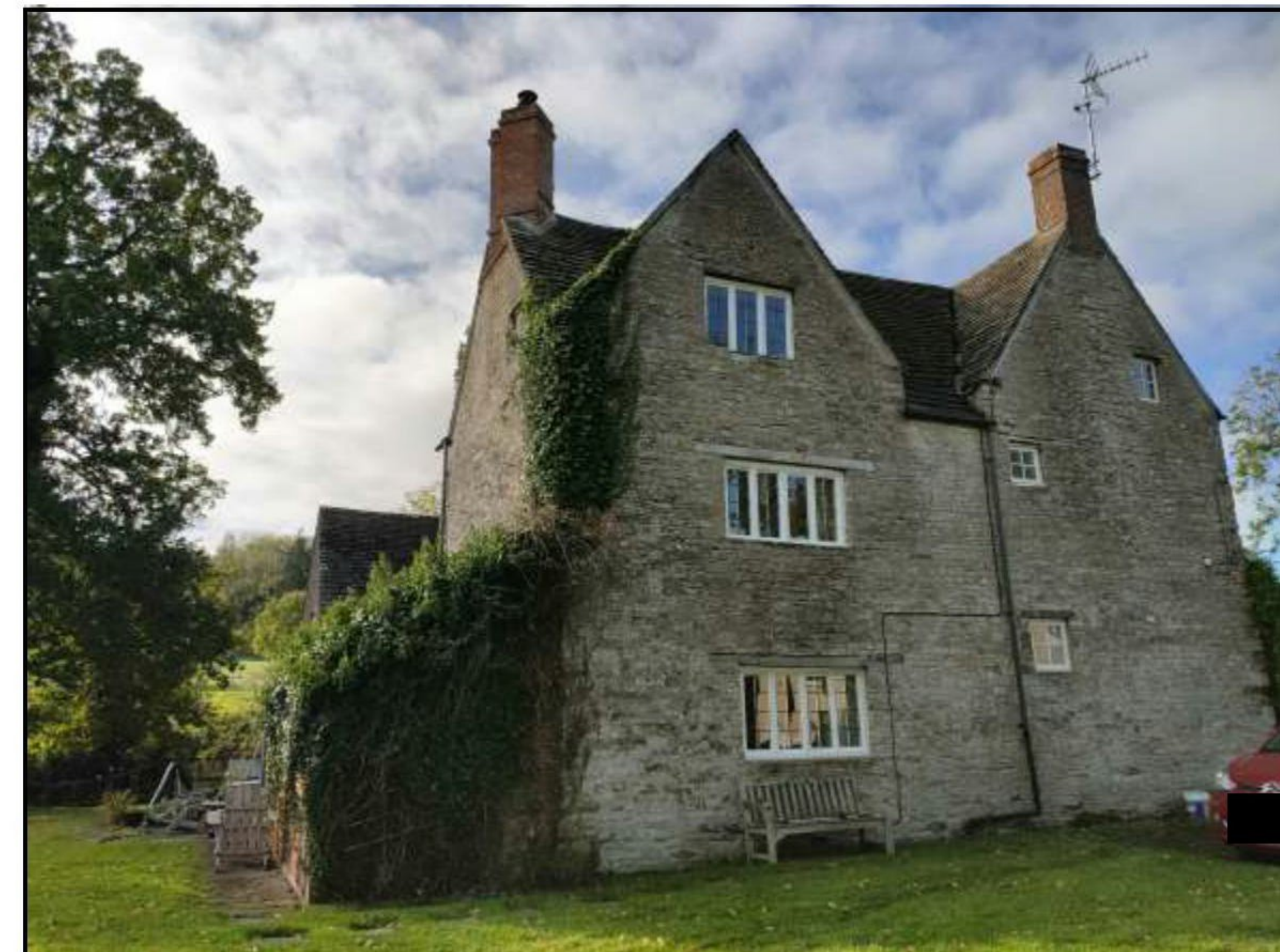
2. Park Gate Cottage; rear/south elevation 3. The east elevation
