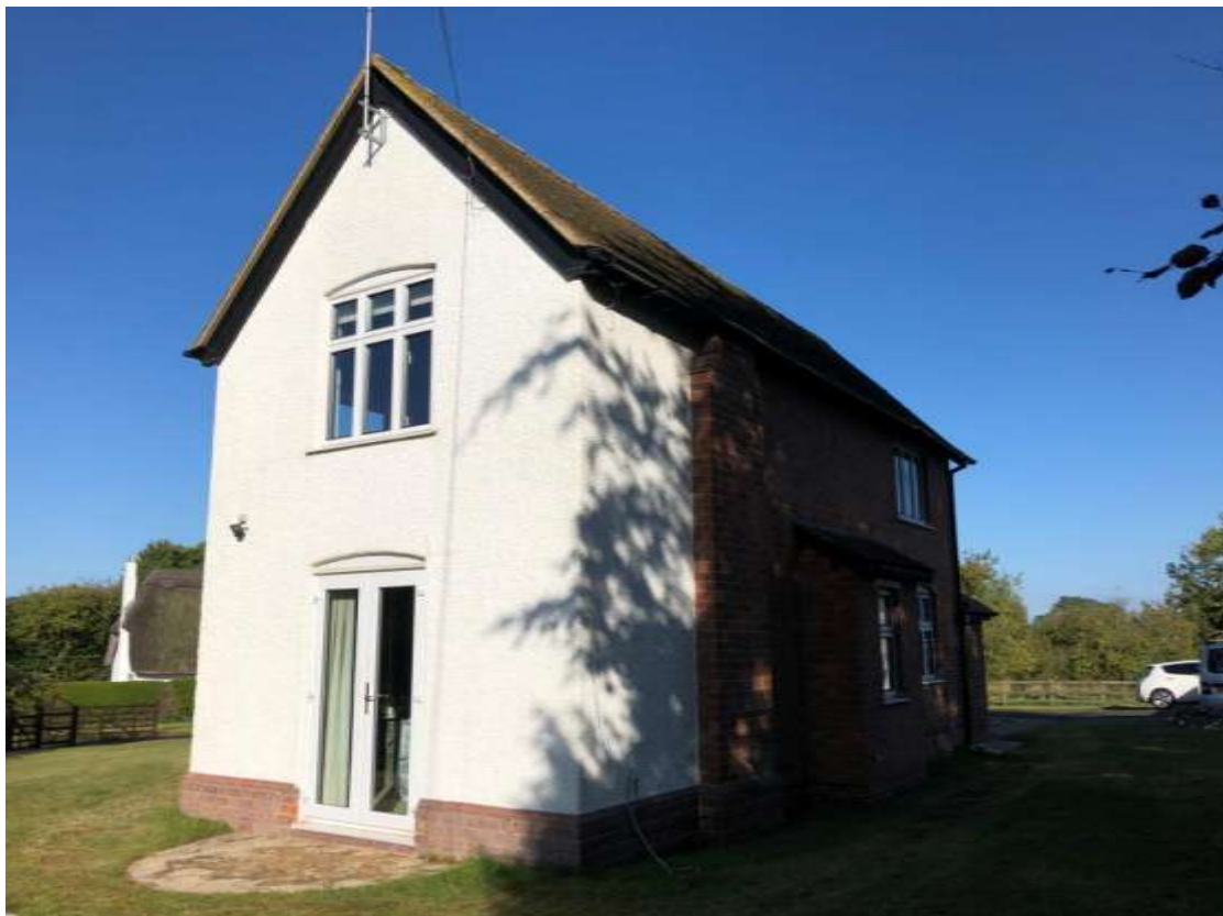
Photo 4 - Side elevation (facing the road) of the existing dwelling.
