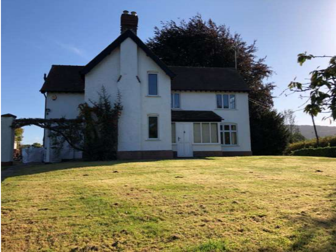
Photo 1 - Front elevation of the existing dwelling.
