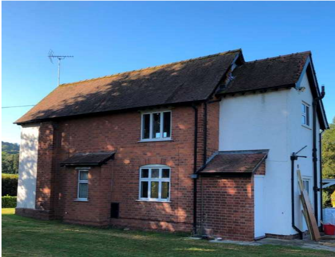
Photo 3 - Rear elevation of the existing dwelling.
