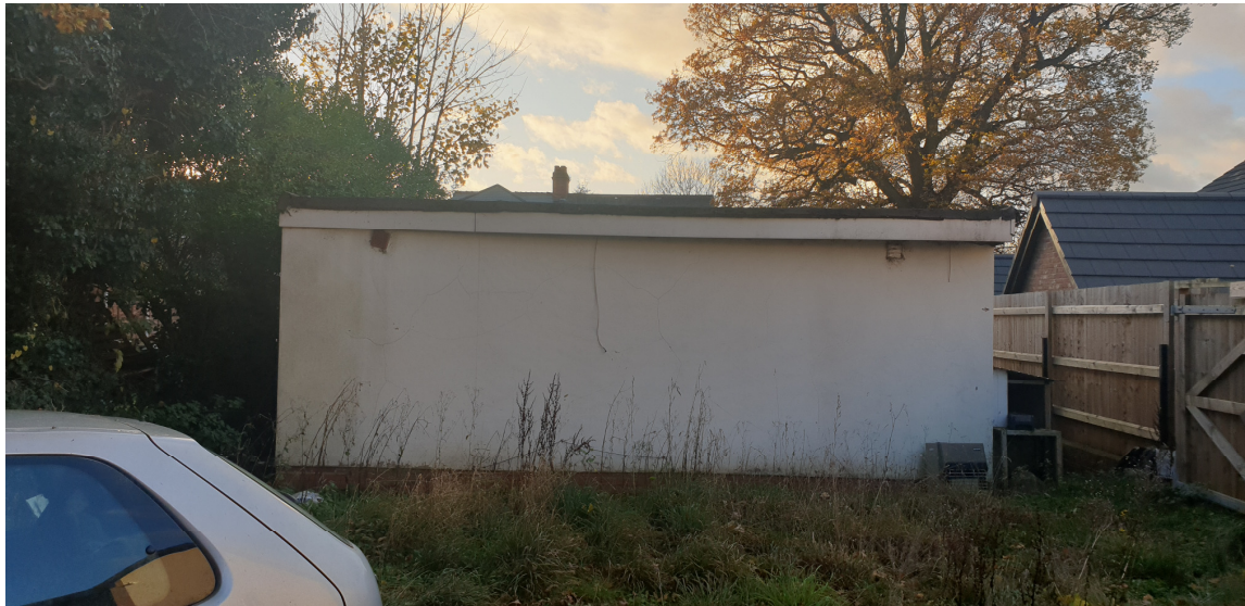
Photo 8 – Rear of garden building No.84
