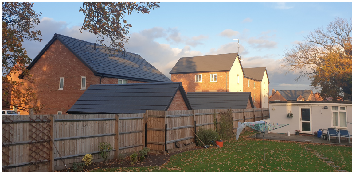
Photo 1a - Looking back from No.84 towards to rear of Old Farm Drive
