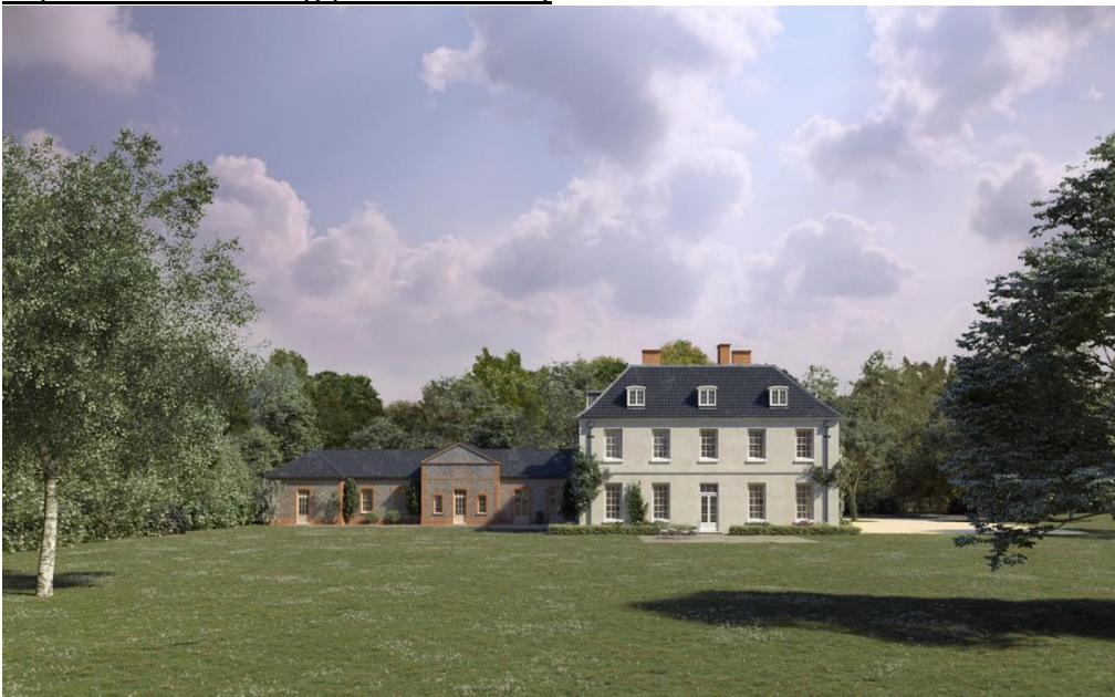
Replacement dwelling (rear elevation)
