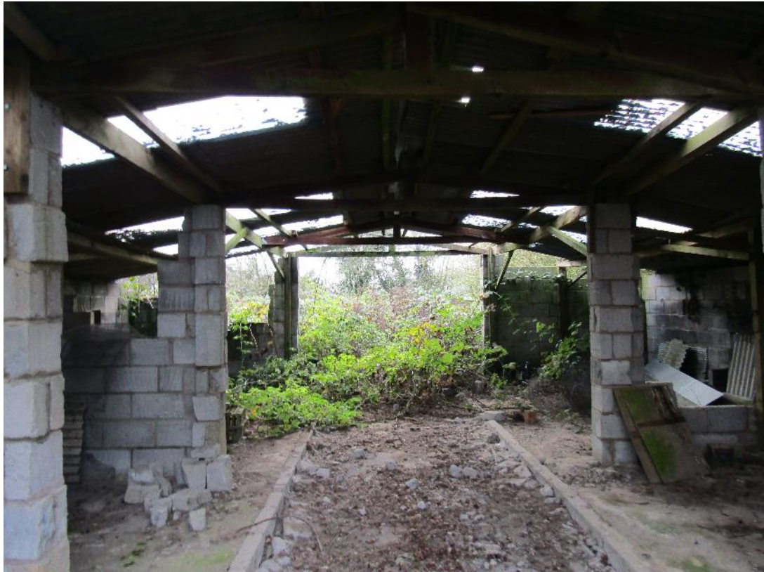
Photo 12 , building three, a breezeblock and corrugated asbestos sheeting construction. Looking south towards the open end of the building which is heavily vegetated with scrub.
