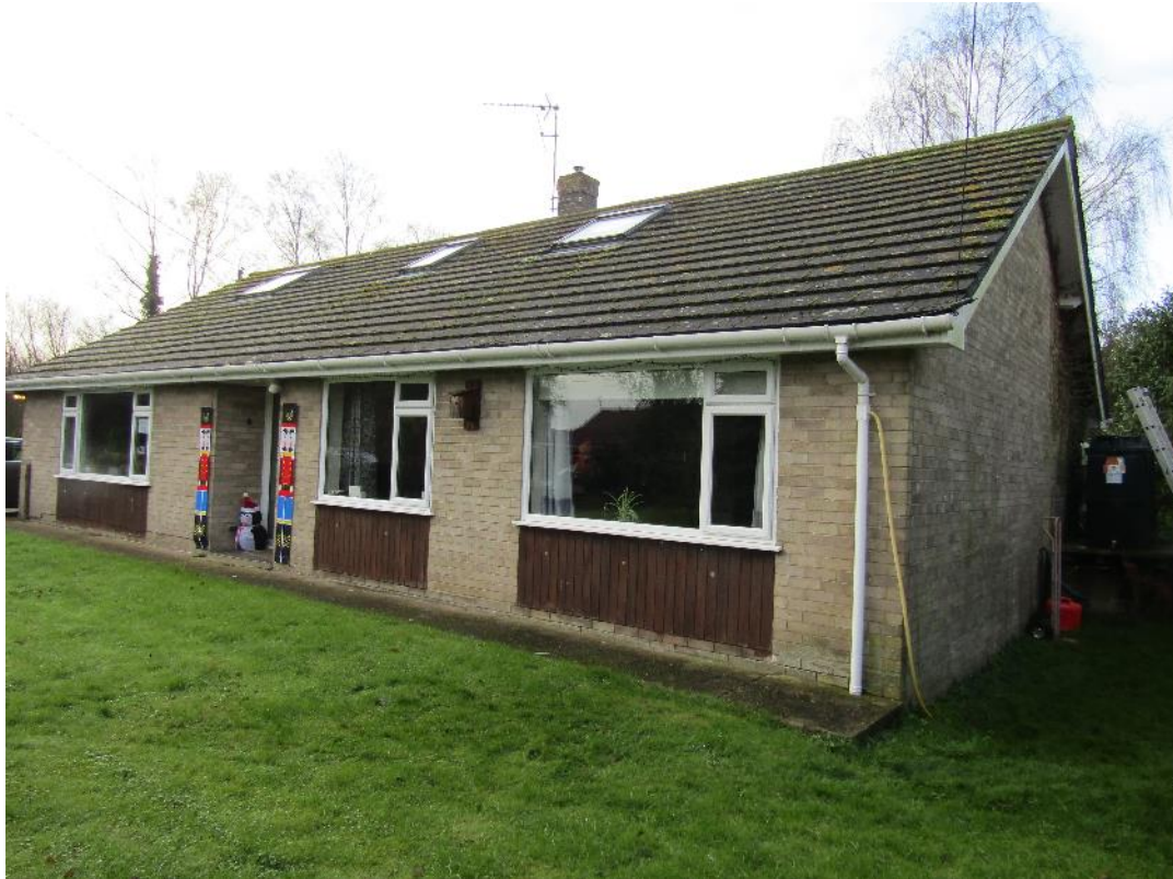
Photo 7 , east and north aspects of the bungalow, looking southwest.
