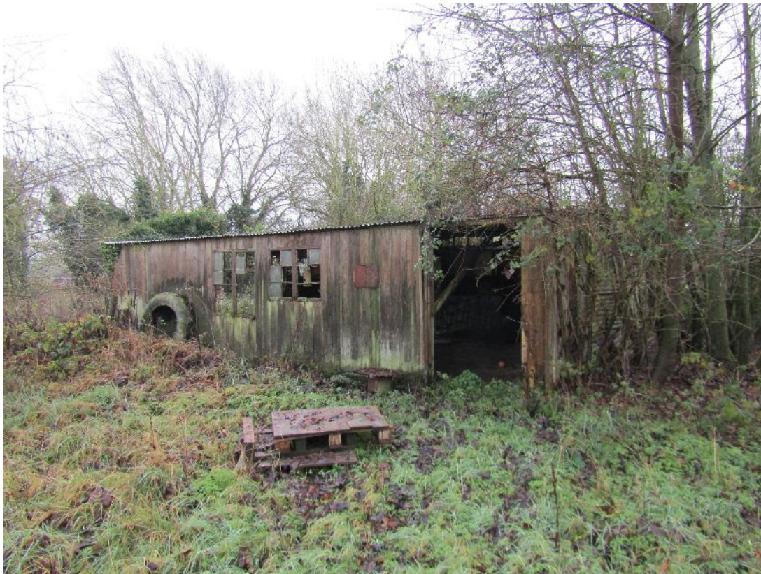
Photo 13 , looking southeast towards building four.
