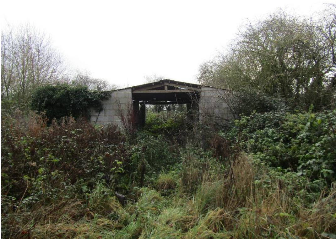
Photo 11 , looking south towards the northern aspect of building three.
