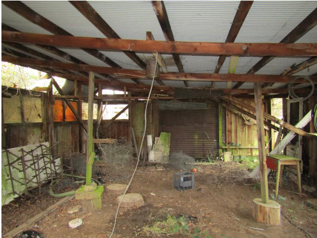
Photo 14 , internal view of building four.
