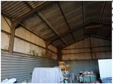
Internally, the vegetation can be seen encroaching in Barn 1 (below) above the horizontal sheeting boards. Portal frame stanchions and raking members are 178x102 UB19, equally divided into 3 bays.
