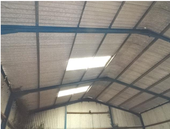
Roof structure and rooflights
