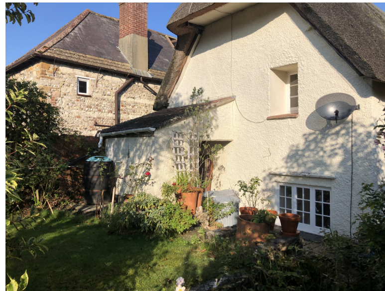
Looking South East
