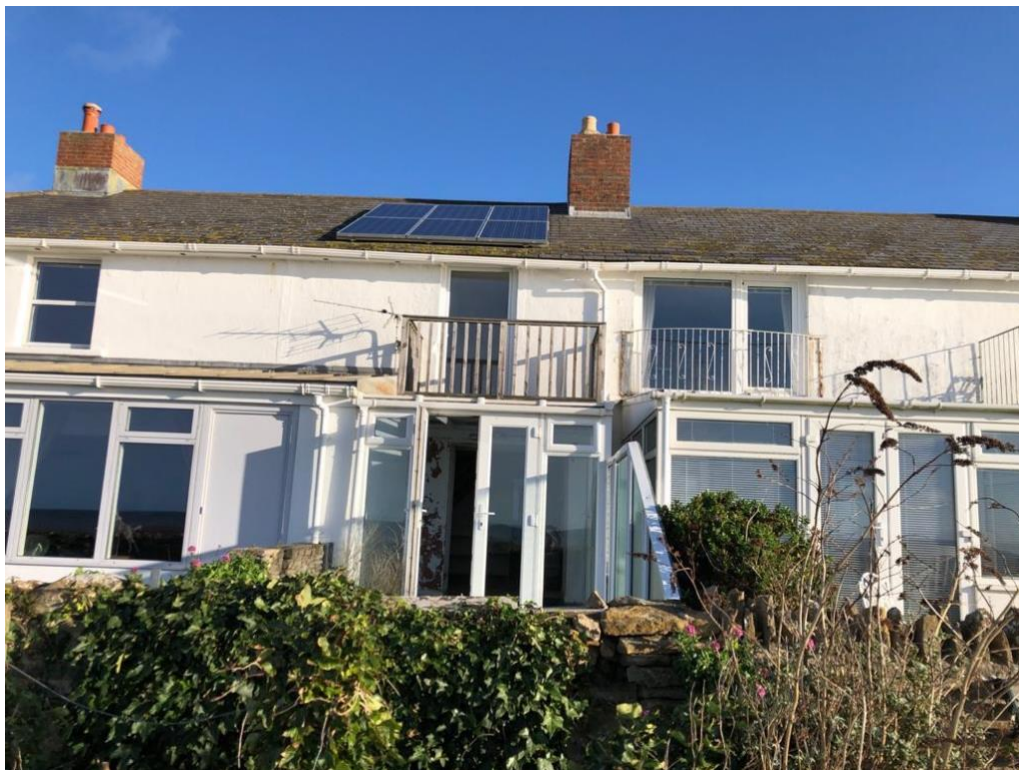
South elevation of 6 Coastguard Cottages
