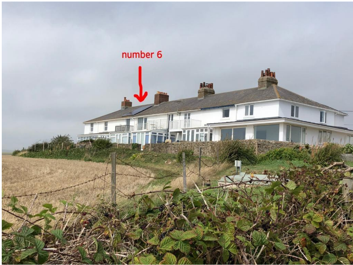
Coastguard Cottages photographed from the south east.
