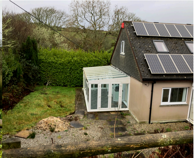
Image 4 – Existing rear (northwest elevation)
