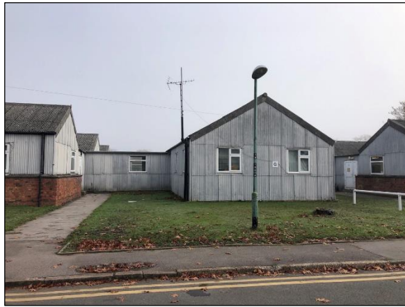
Photo 1: Type B gable end with C link to A
