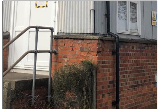
Photo 13: Flaking brickwork
