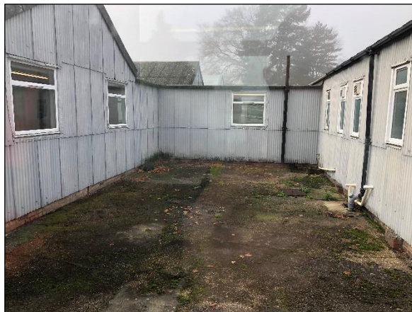
Photo 3: Enclosed concrete courtyard
