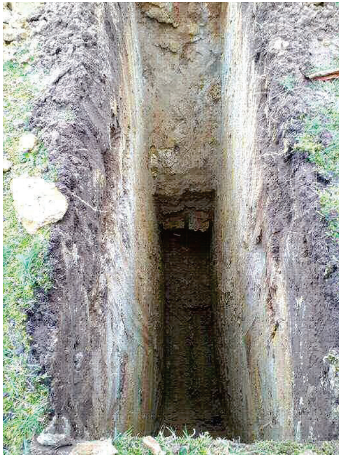
Photograph 6: View of TP02.
