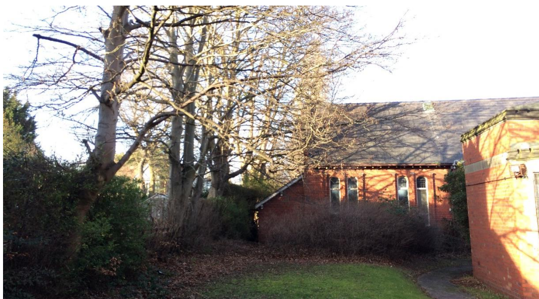
Figure 2 View north showing trees along western boundary growing adjacent or close to the church.
