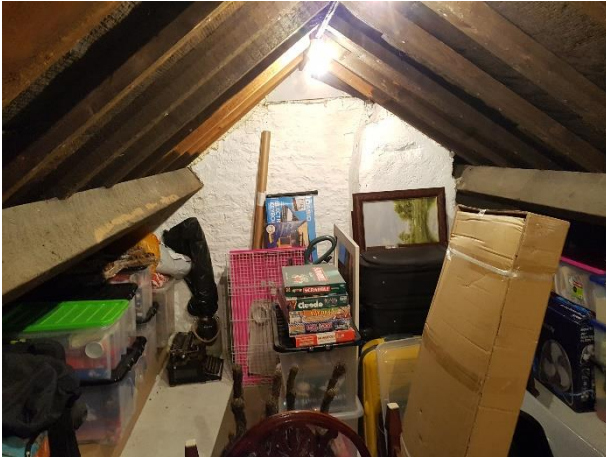
Photograph 7. Southern interior of the eastern wing, with bitumen and mineral underlay and simple timber frame.
