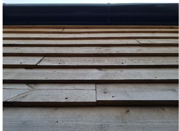
Photograph 8. Tight-fitting timber weatherboarding on the eastern wing.
