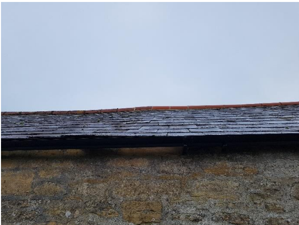
Photograph 9. Tight-fitting slate tiles of the eastern wing.
