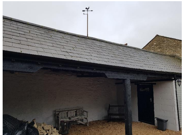
Photograph 4. Open-sided western wing of the dwelling.
