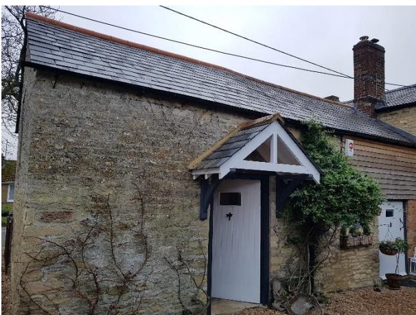
Photograph 5. The eastern wing of the dwelling, viewed from the west.
