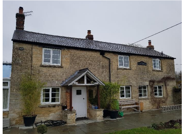
Photograph 2. The dwelling viewed from the south-east.
