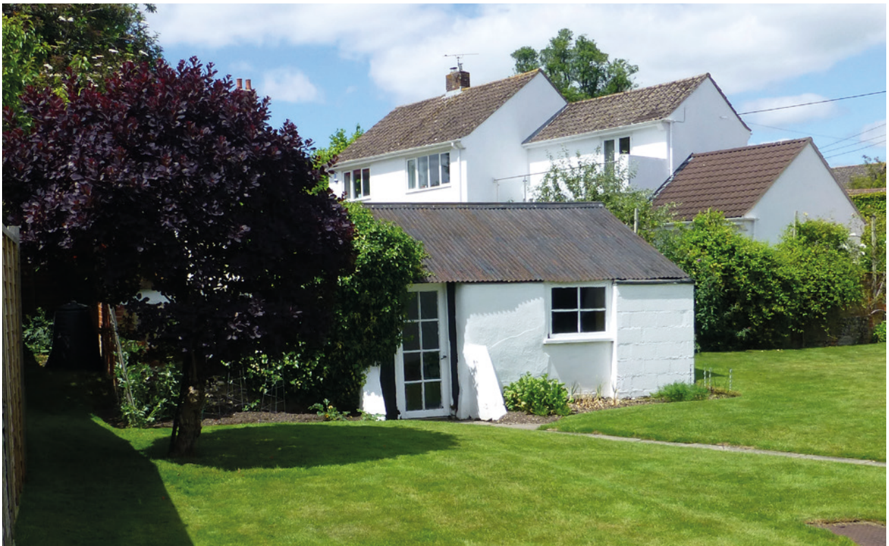
View of existing outhouse from south.
