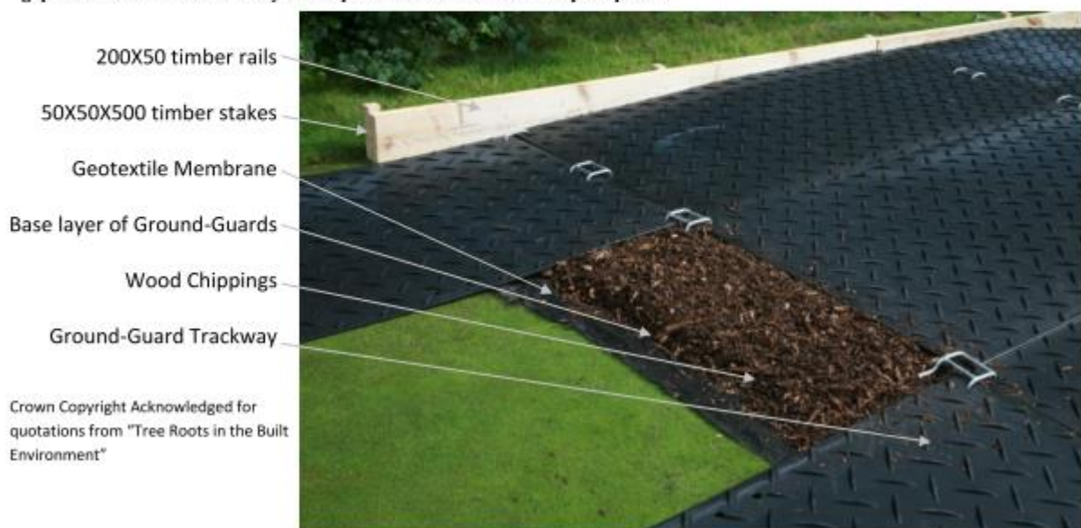
Ground-Guard trackways should have additional cushioning installed where they pass near to trees.
