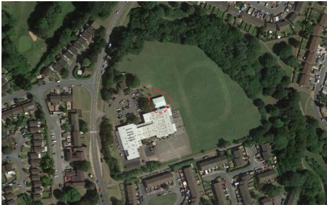
Aerial view of Glyncoed Primary School. Circled area shows existing unit to be removed.
