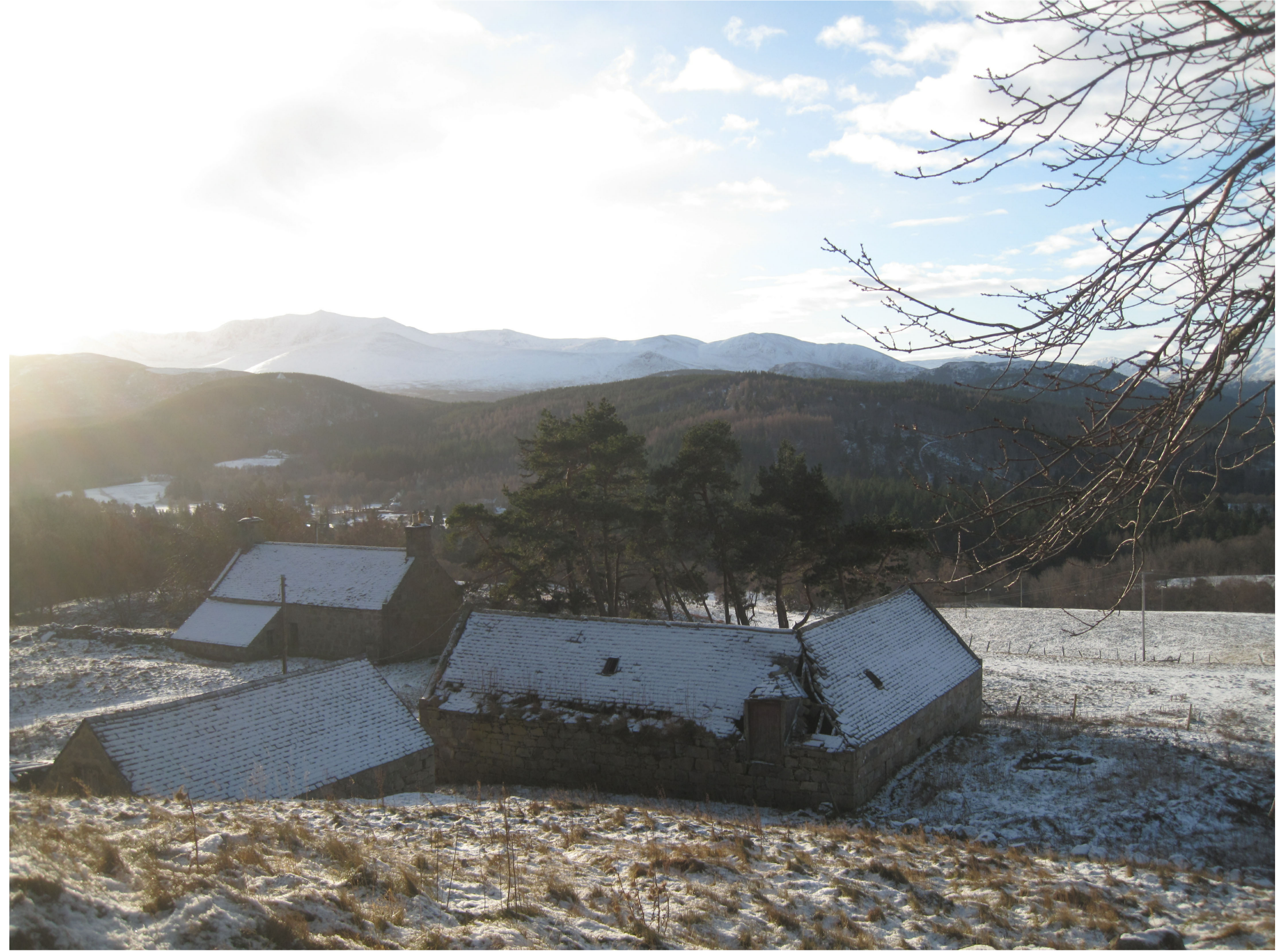
Taken 18.01.2011 North West corner Overview of Steading, Farmhouse & Steading B, prior to roof collapse
