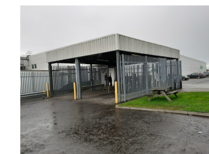
Existing Car Park - Photograph P1
