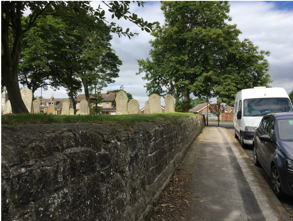
Plate 9 View of northern graveyard boundary wall of the Church of St. John illustrating the level difference between the graveyard and the road
