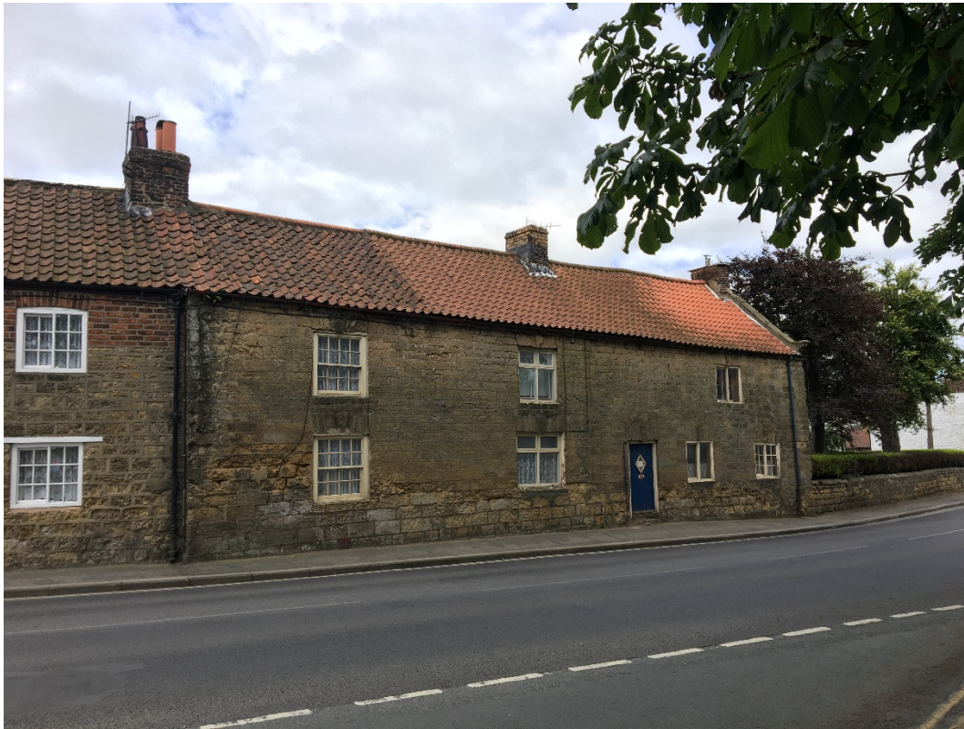
Plate 17 82, 84 Main Street, grade II listed – within Conservation Area – vertical sash on this building with flat arches with keystones. The kneelers survive on the gable
