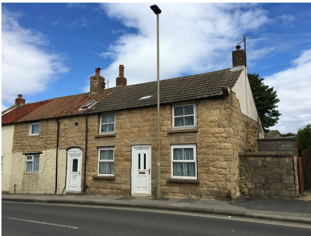
Plate 20 Even buildings which have been substantially repaired and altered retain the curved kneelers
