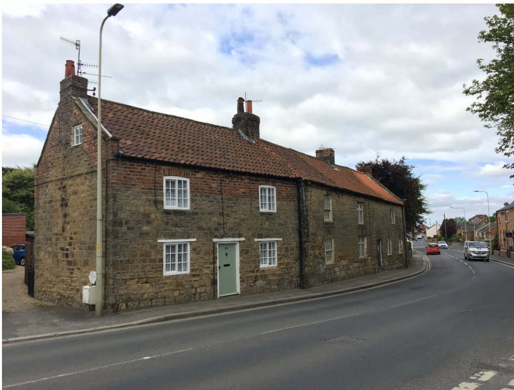
Plate 16 Grade II listed 86 Main Street and Grade II listed 82, 84 Main Street in Conservation Area – note the coped gables, sandstone, pantiles and horizontal sash.
