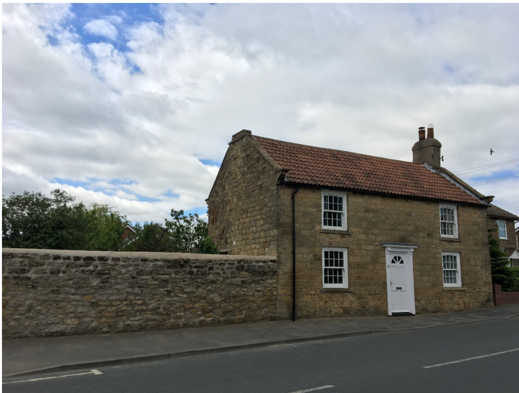
Plate 18 Historic building on Cayton Main Street – curved kneelers evident along with vertical sash windows, pantile roofs and upper floor openings just below the eaves
