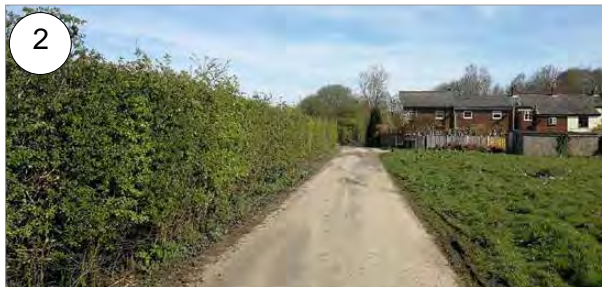
2 Existing access to old engine cottage
