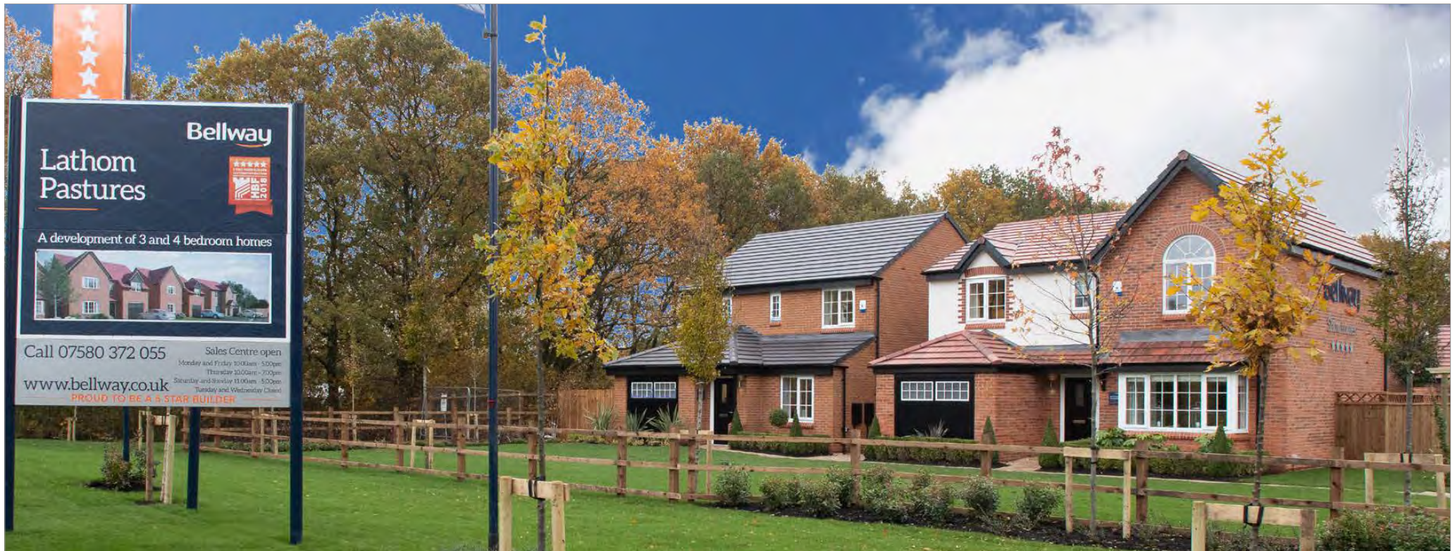
Figure 1 - Phase 1 under construction
