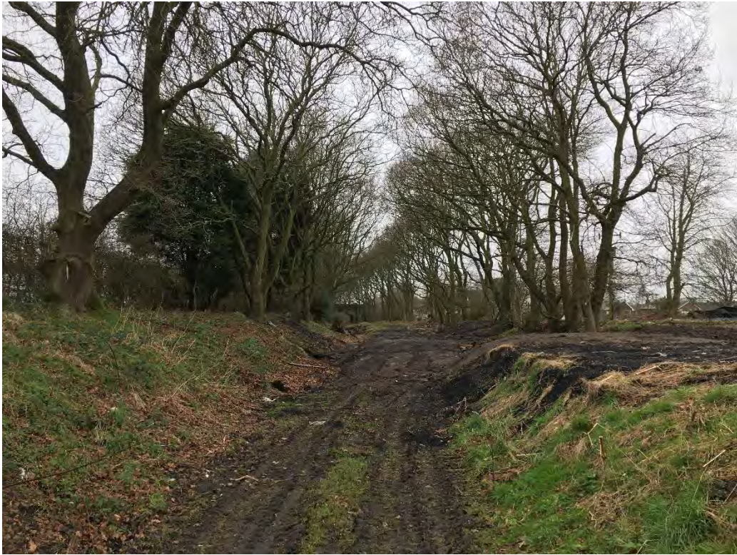
Plate 1: View west looking at disused railway track with bridge shown in background
