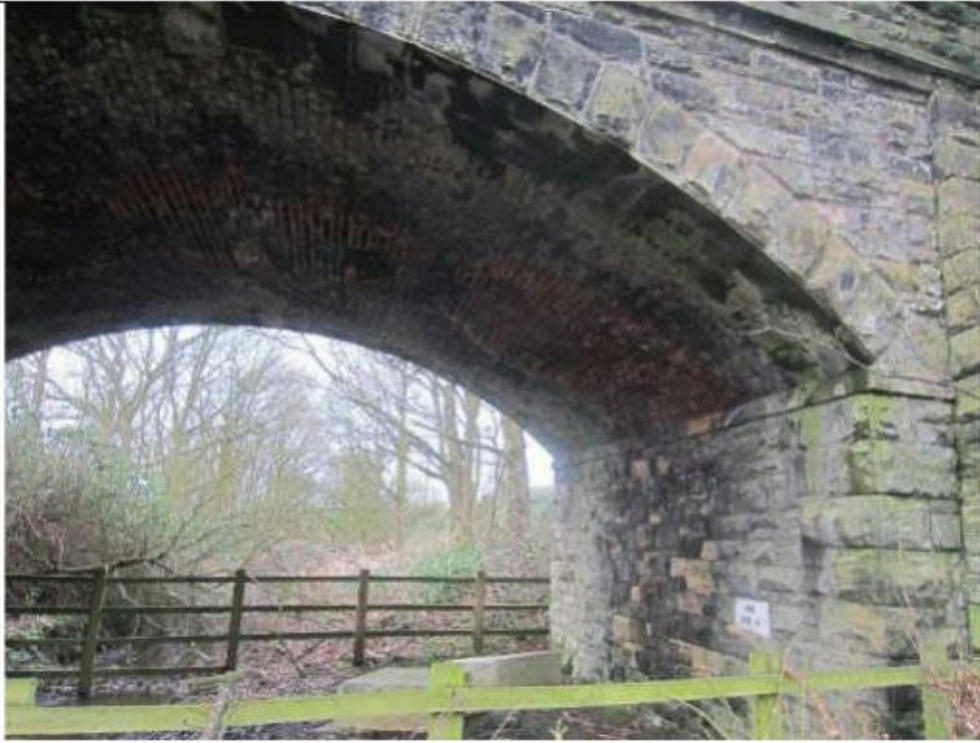
Photo 37: Firwood Road bridge at western end of disused railway corridor (west)
