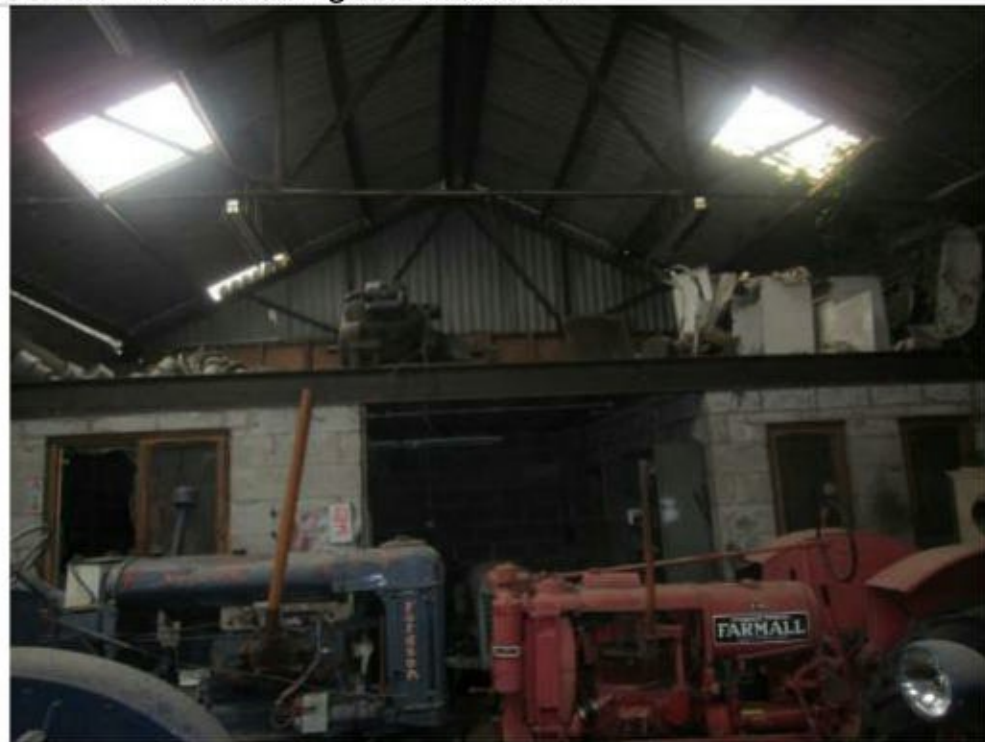
Photo 27: Interior of B1 showing skylights
