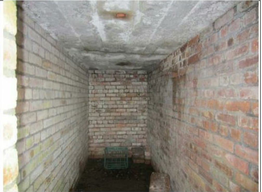
Photo 32: Interior of B4
