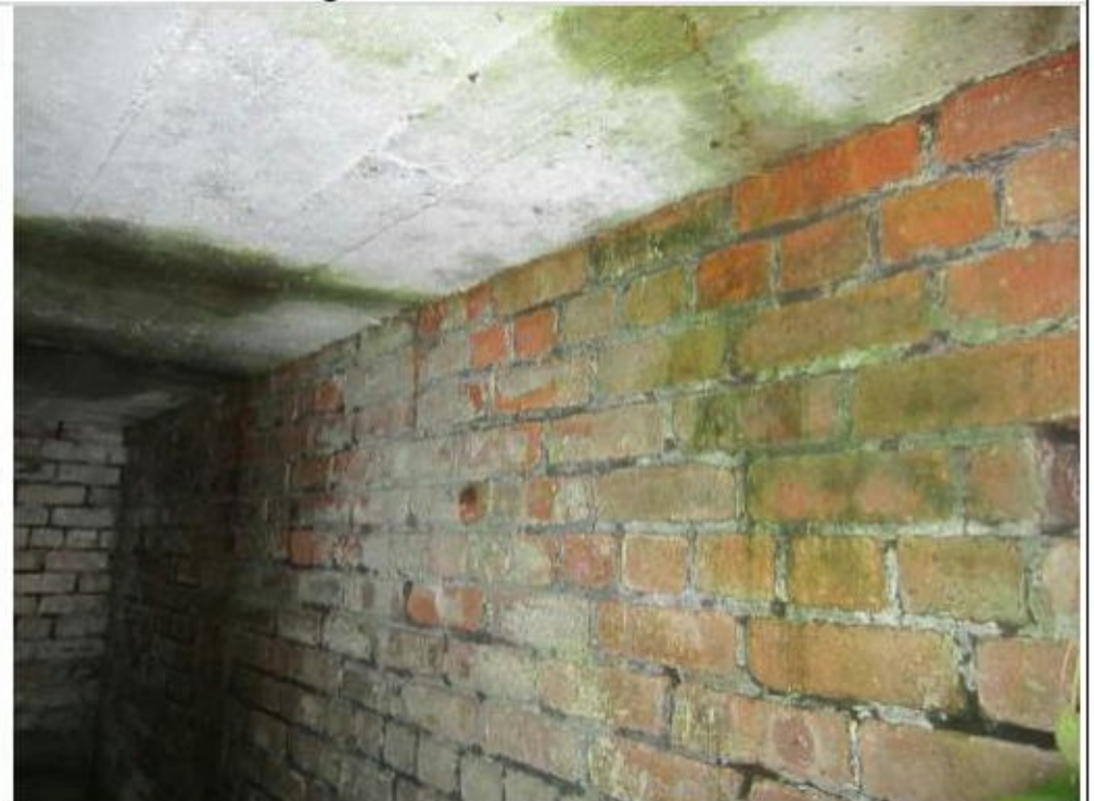
Photo 30: Interior of B2
