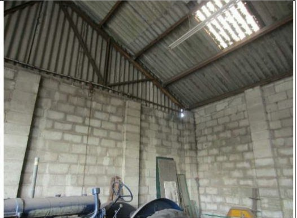
Photo 26: Interior of B1 showing skylights
