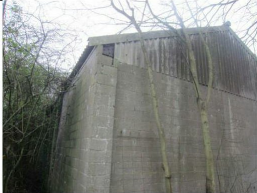
Photo 25: Western gable end of B1
