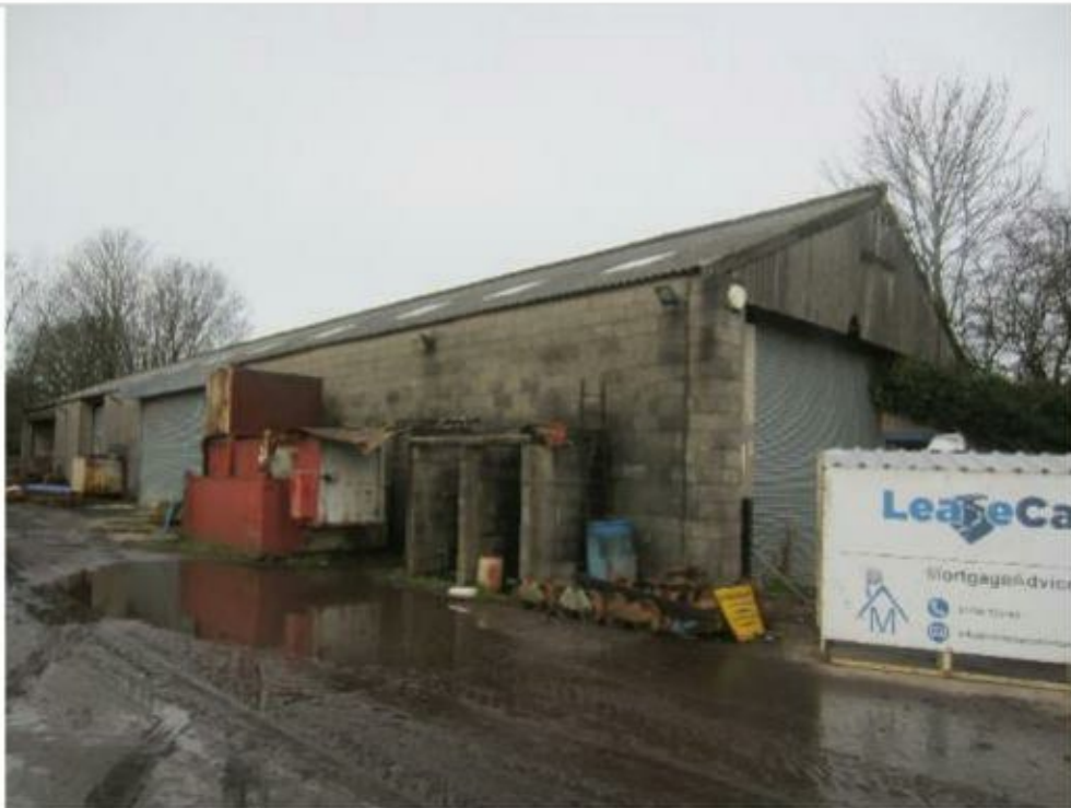
Photo 23: Southern and eastern elevations of B1
