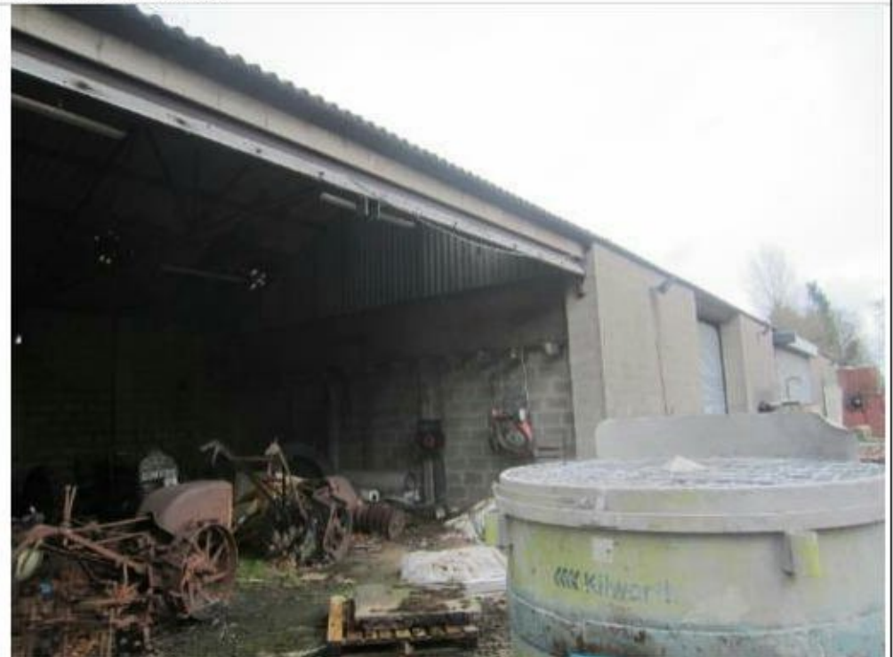
Photo 24: Western end of B1
